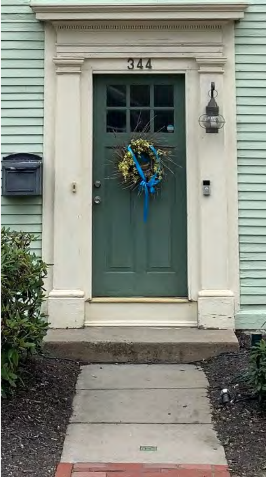
Figure 5 – Walkway Preservation and Step Replacement
