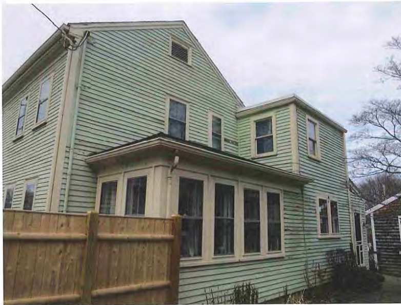
17_View north showing southeast elevation from west end
