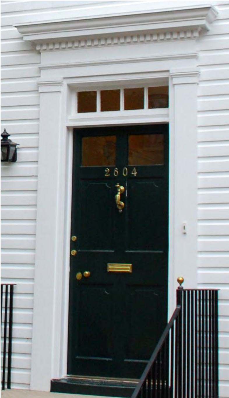
Figure 3 – Example Federal-Style Door Replacement
