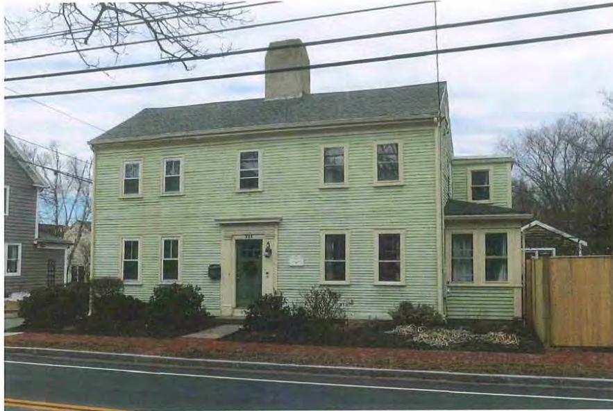
5_View northeast showing principal facade (southwest elevation)
