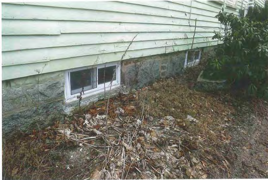
16_View southwest showing northeast elevation - detail of foundation to ell and basement windows
