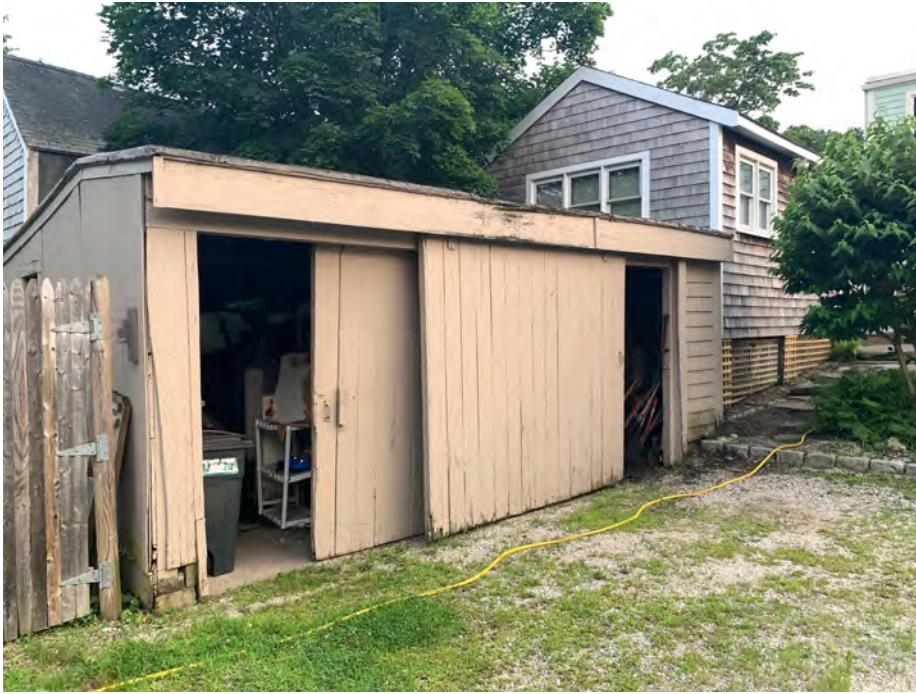
Figure 10 – Rear Shed to be Removed
