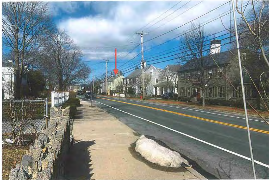
1_ Setting - View northwest along Merrimac Street showing Carr House (center) and neighboring houses on northeast side of the street
