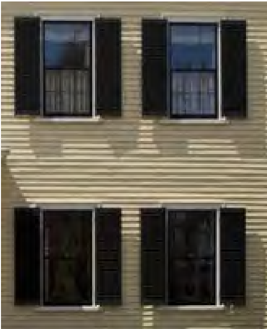
Figure 6 – Example of Federal-Style Shutters
