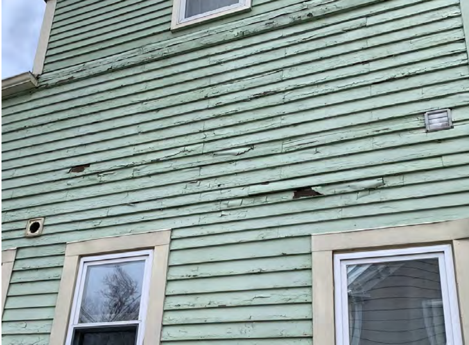
Figure 8B – Clapboard Repair
