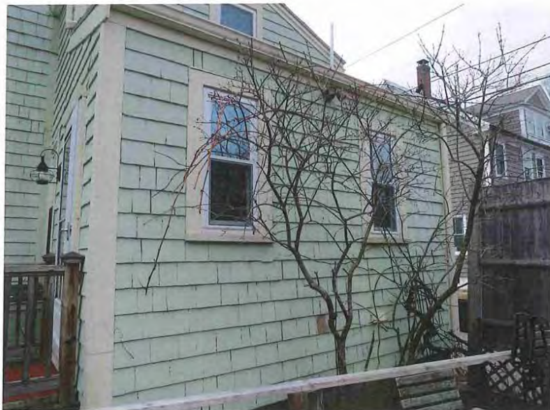
23_View northwest at rear (southeast) elevation - detail of northeast addition
