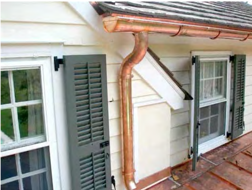
Figure 7 – Examples of Gutters and Downspouts
