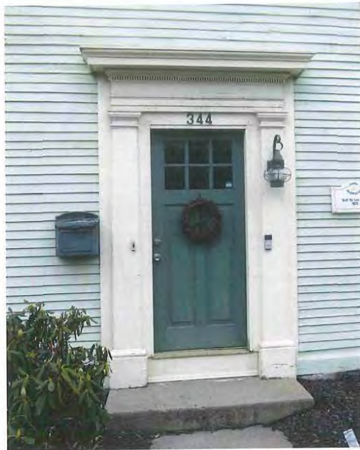
9_View northeast showing principal facade (northwest elevation) - detail of main entry
