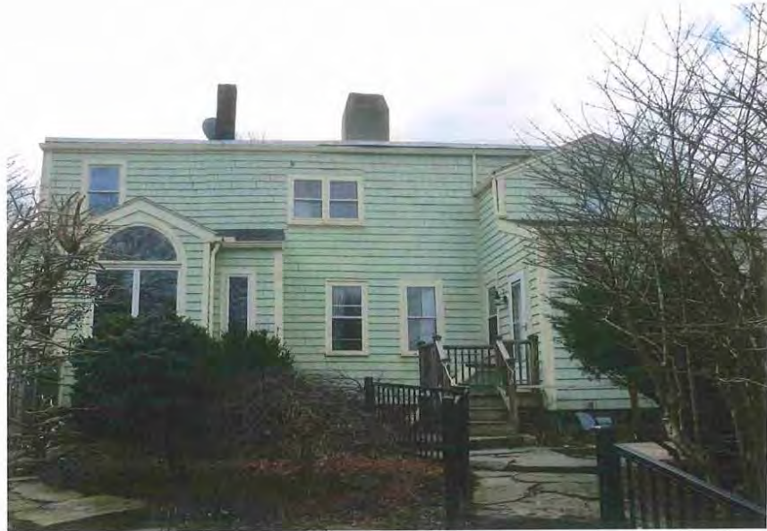
22_View southwest showing rear (southeast) elevation
