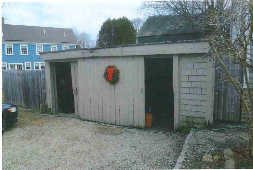
30_View southeast showing northwest elevation of shed
