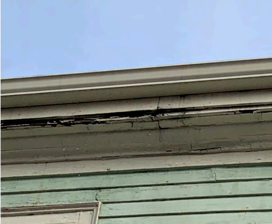
Figure 8A – Soffit and Trim Repair
