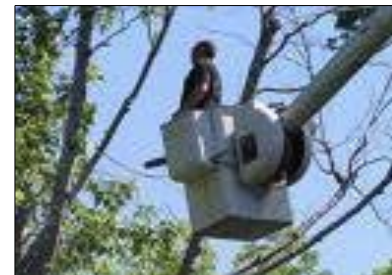
Tree-pruning to Protect Utility Lines
