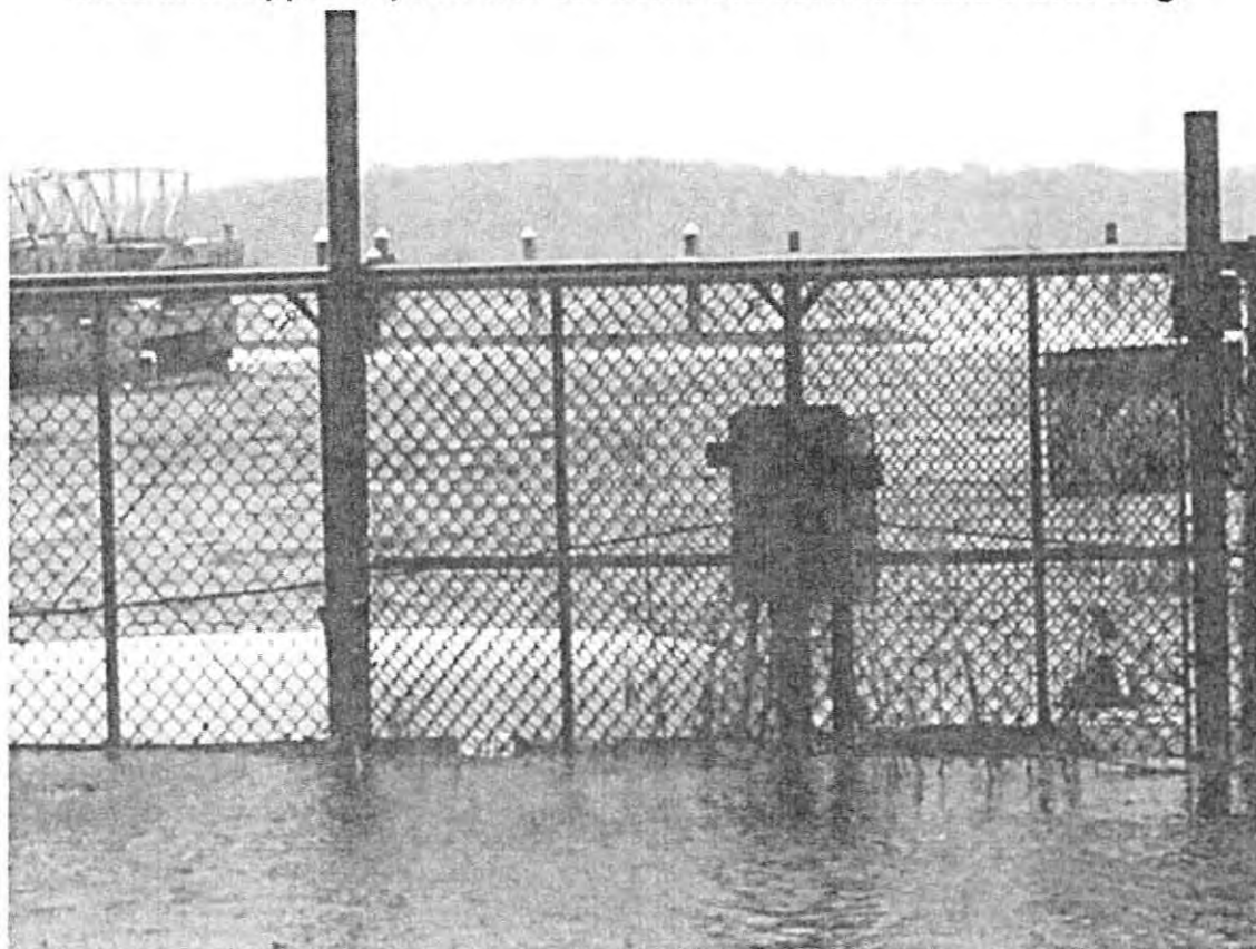
Storm surge flooding (May 2018)
