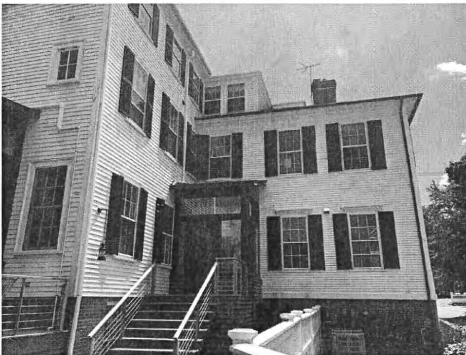
Photo 6, Main House, North Elevation, July 2019
