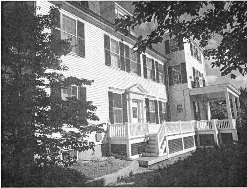
Photo 3, Main House, East Elevation, July 2020
