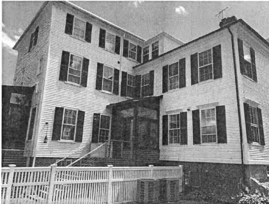
Photo 7, Main House, South West Elevation, July 2019
