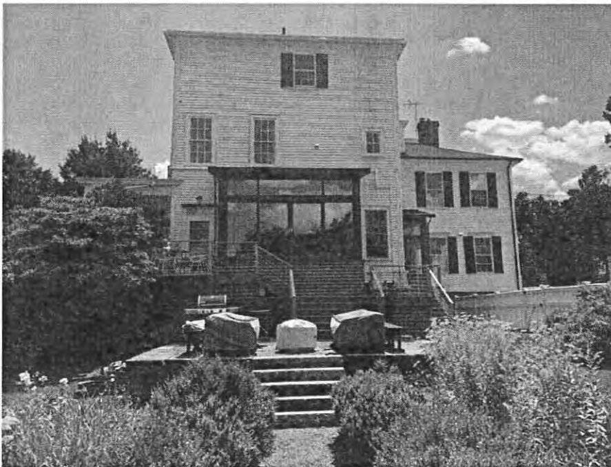
Photo 7, Main House, South Elevation, July 2019
