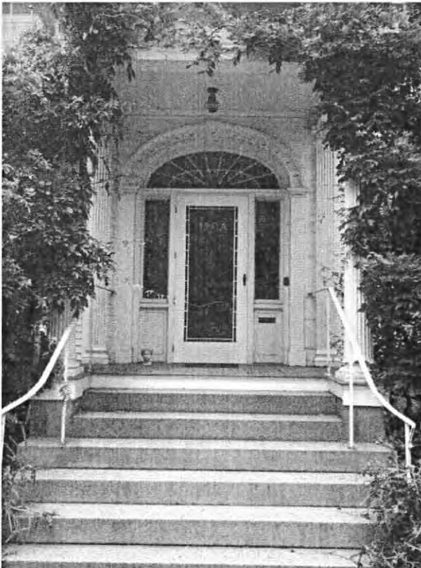
Photo 2, Main House, South Elevation, July 2019
