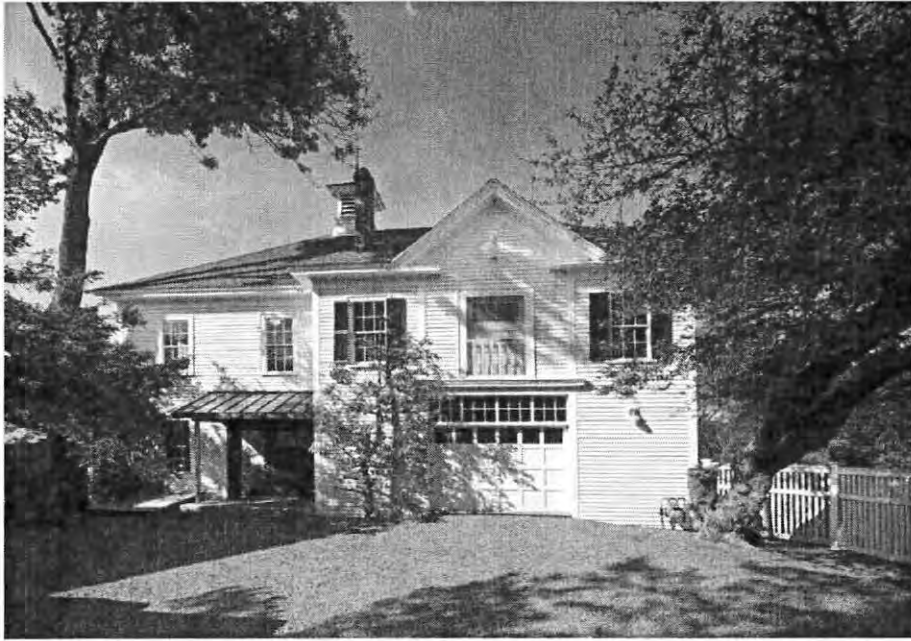
Photo 8, Carriage House, South Elevation, July 2019
