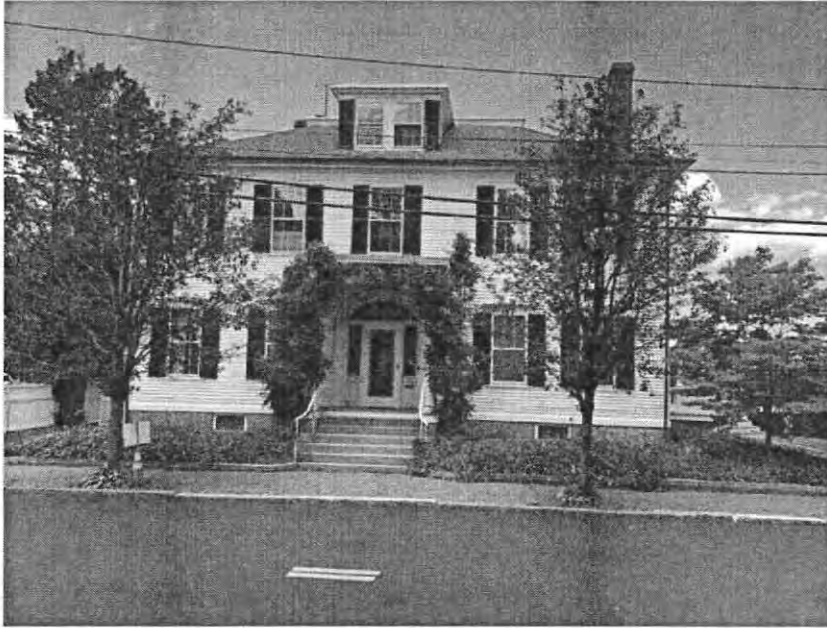
Photo 1, Main House, South Elevation, July 2019
