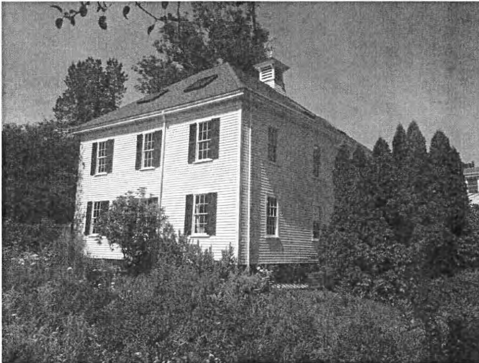
Photo 12, Carriage House, North East Corner, July 2019
