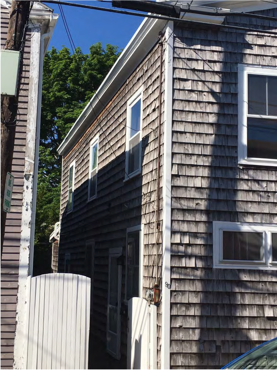
Photo B East Facade
