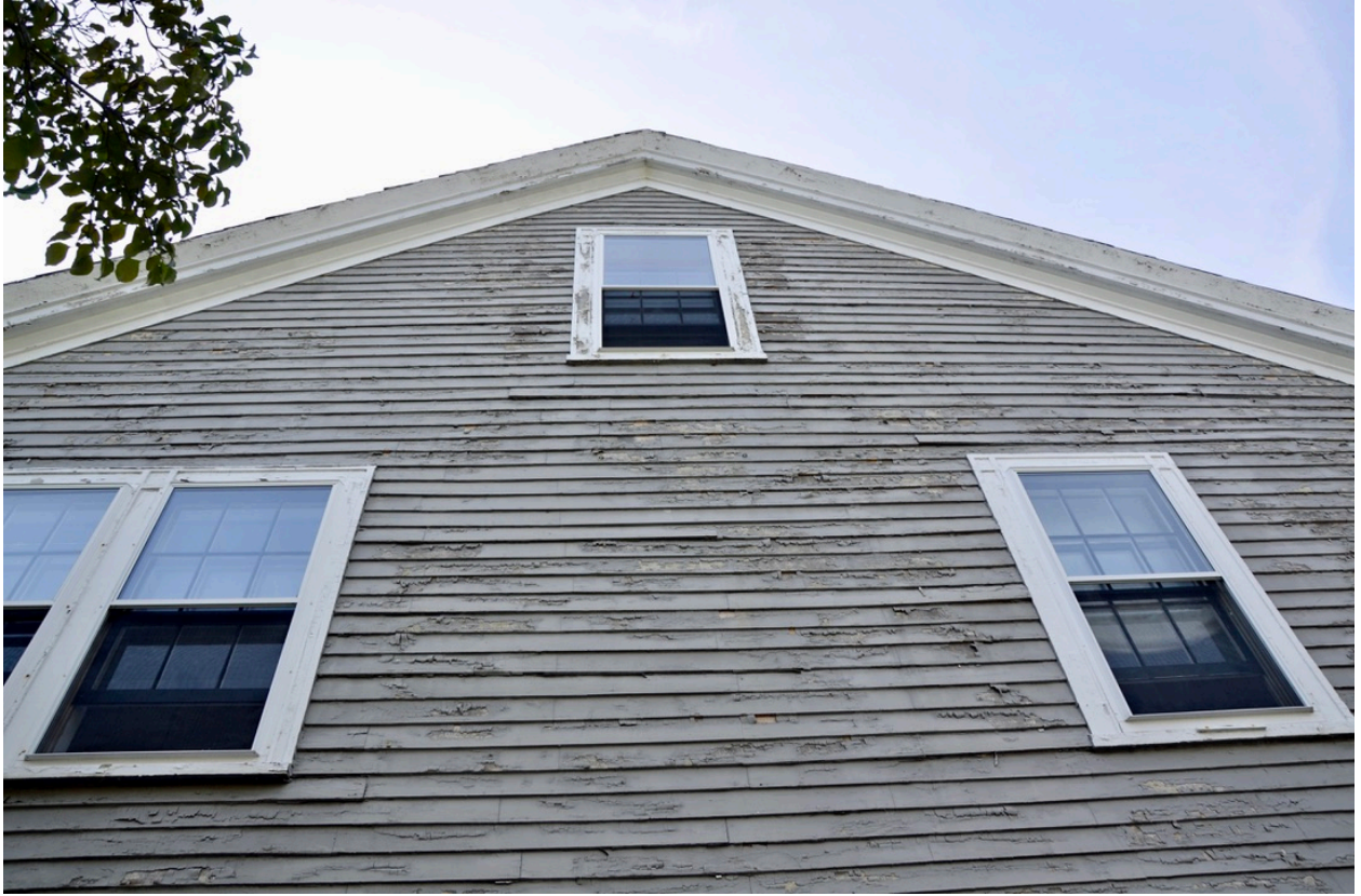
10. West Façade Windows, Trim, Siding and Rake Details.
