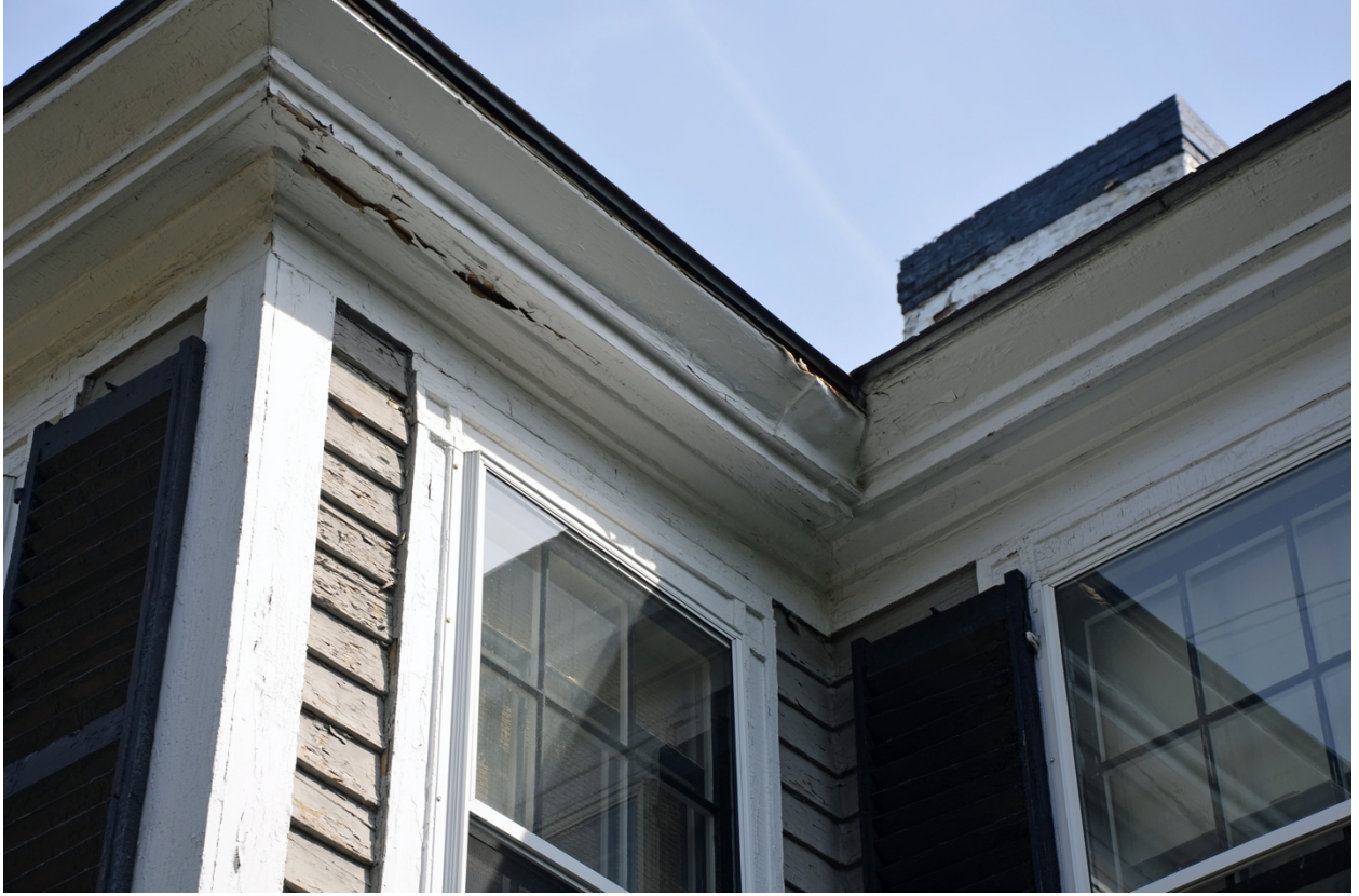
5. Fascia, Crown, Soffit, Frieze and Casing Detail
