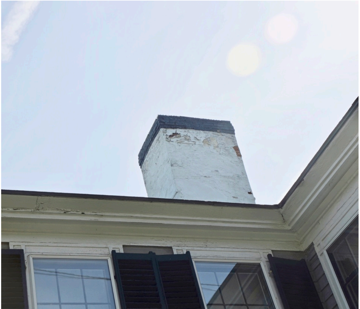
6. Fascia, Crown, Soffit, Frieze and Chimney Detail
