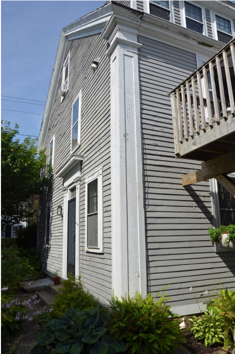
12. Corner Pilaster, Rake, Fascia and Return Detail
