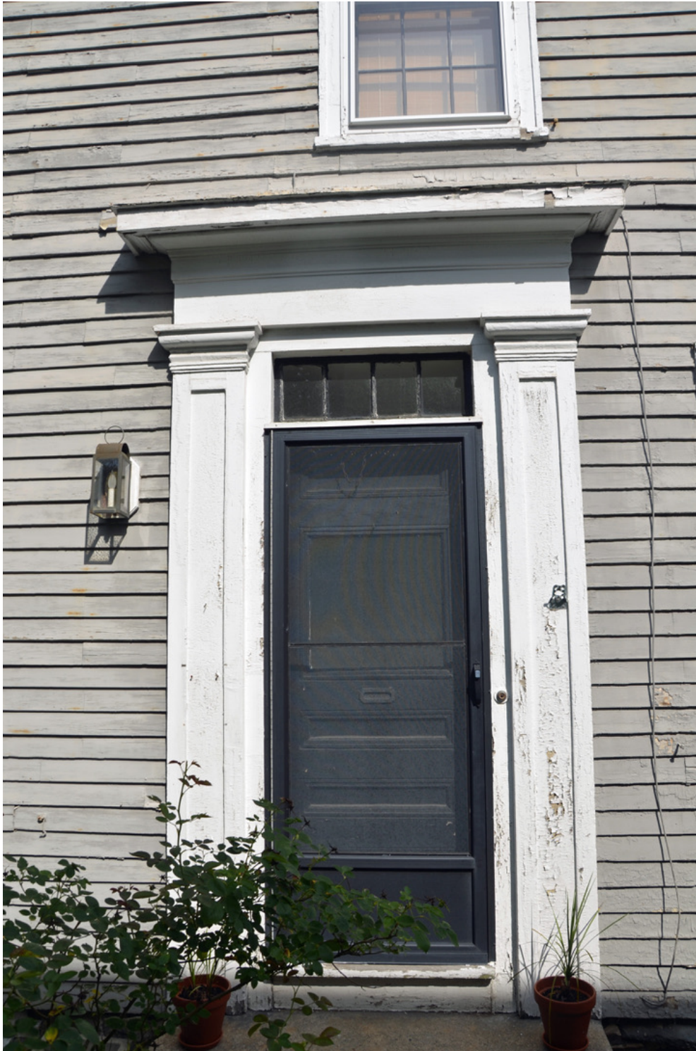
11. East Entry Door with Transom Window, Pilasters, Frieze, and Cornice Detail.
