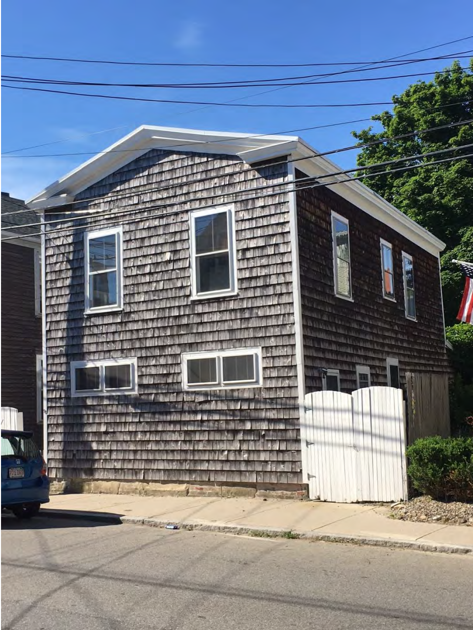
Photo D North Façade On Water Street
