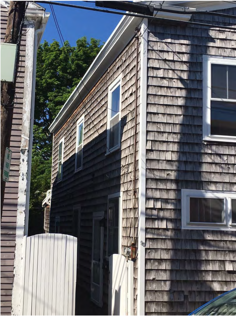
Photo B East Facade
