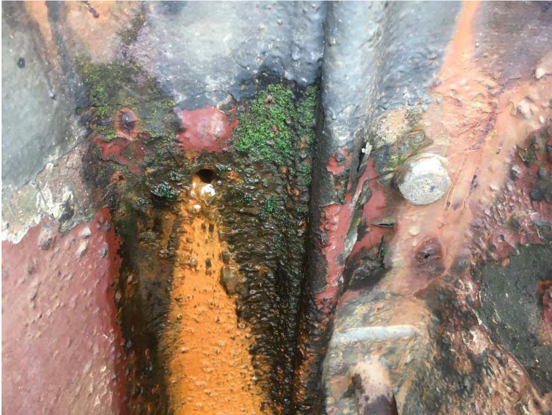
Missing Tie Back Anchor Bolts
