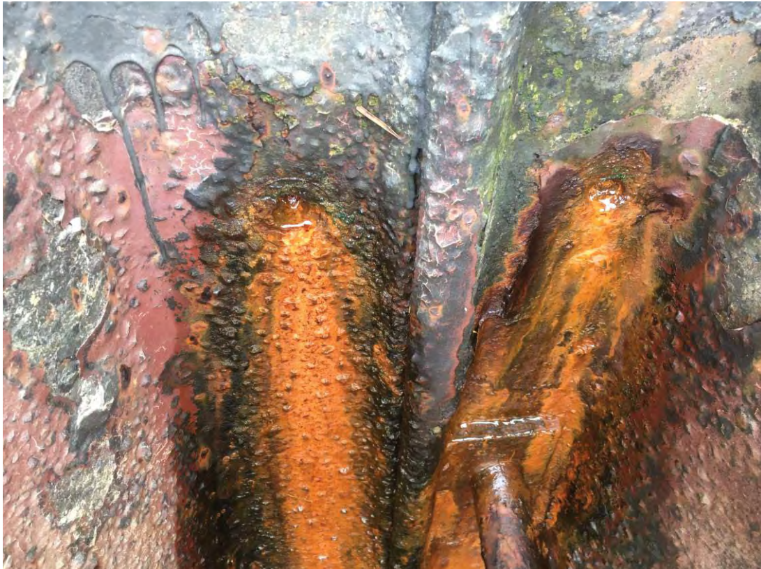
Missing Tie Back Anchor Bolts
