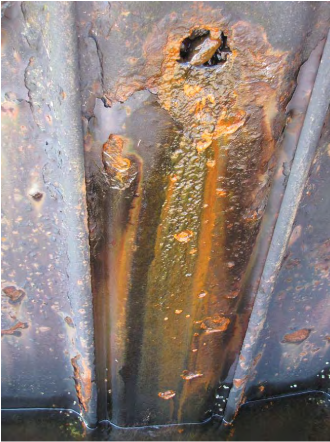
2013 typical conditions: corroding weep hole
