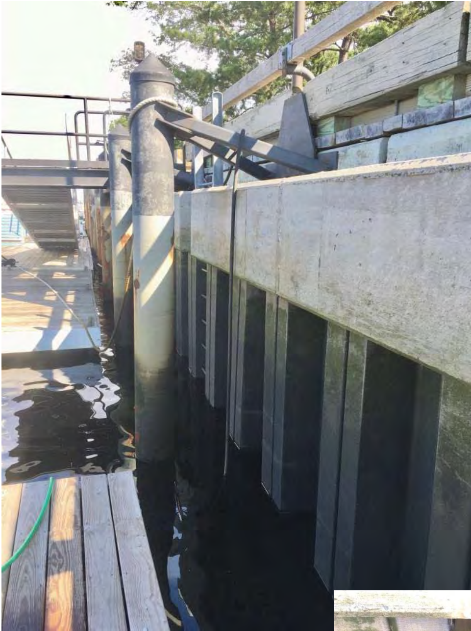
FRP sheet piles with concrete infill and mooring pilings
