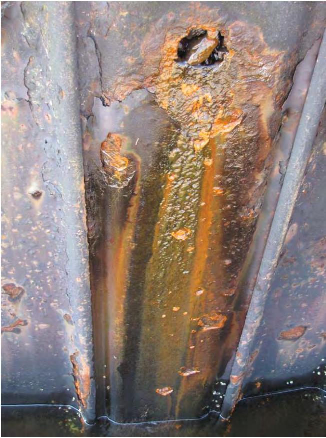
2013 typical conditions: corroding weep hole
