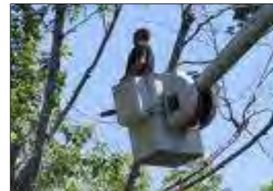
Tree-pruning to Protect Utility Lines
