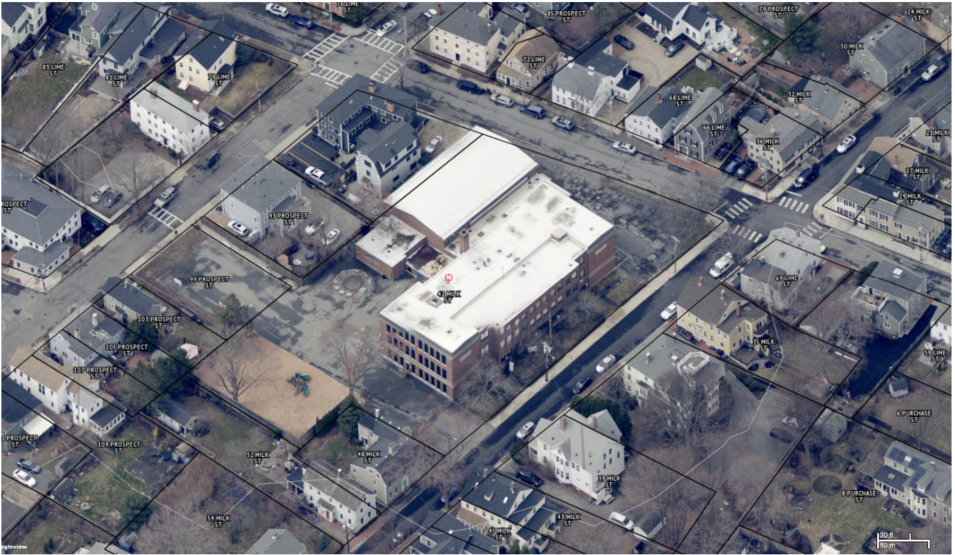
Brown School Property – View from East
