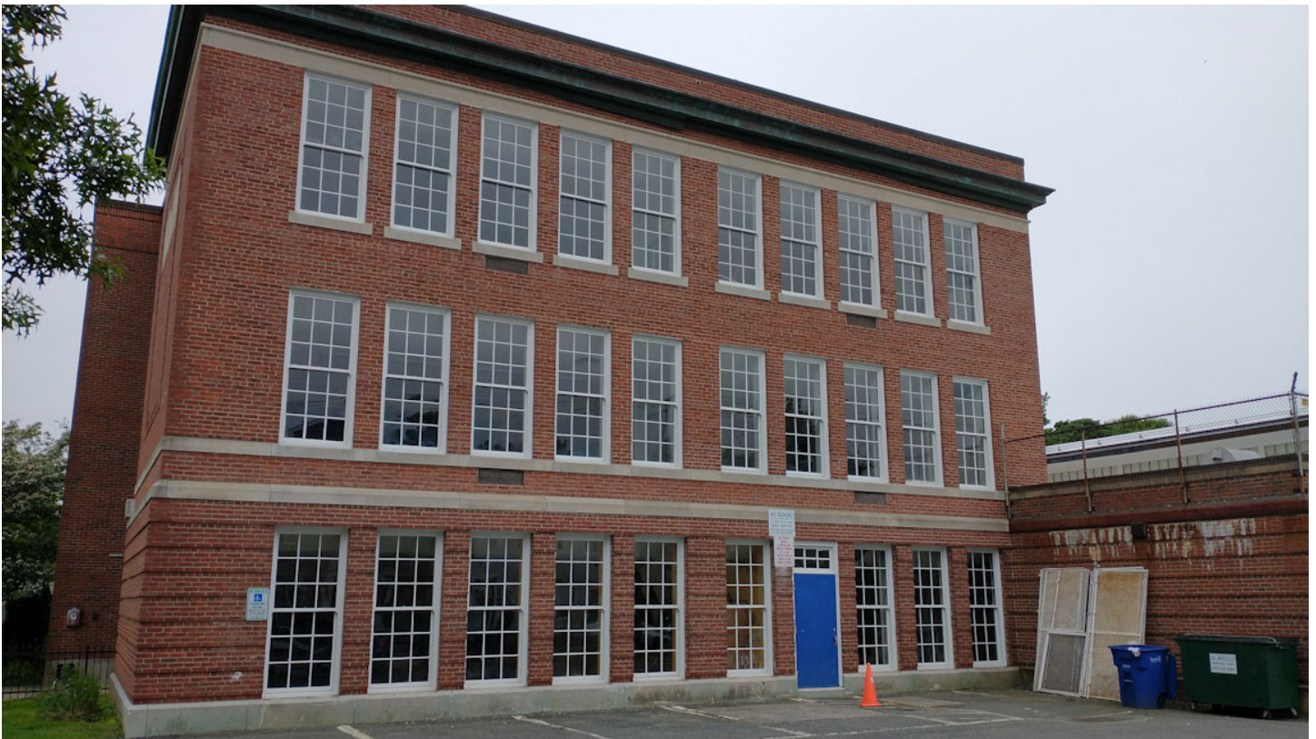
Former Brown School – Main Building – Partial Window Renovations Completed in 2022
