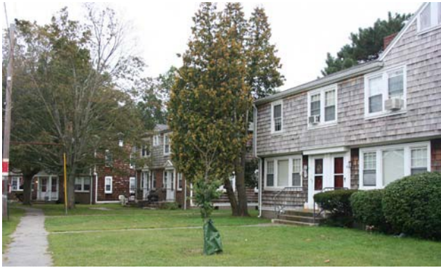
Newburyport Housing Authority Family Housing
