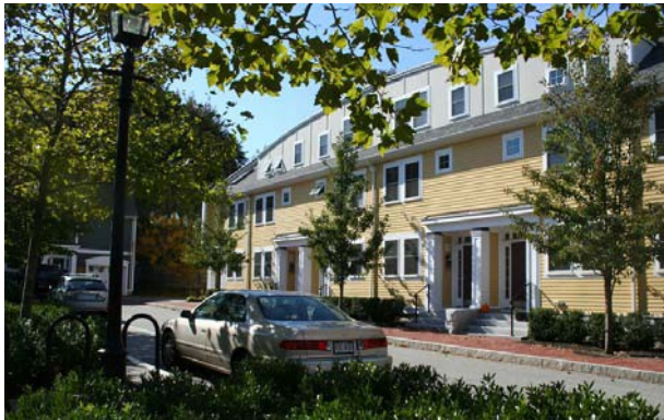
Foundry Square - Merrimack Street Multi-family
