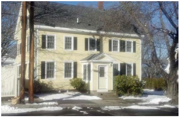
12-14 Woodland Street Affordable Rehabilitation
