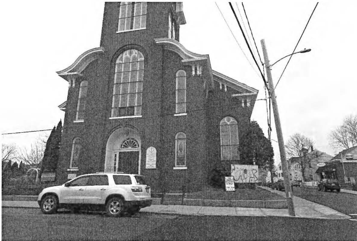
Photo 8. East Elevation, 1861 Portion, January 2020
