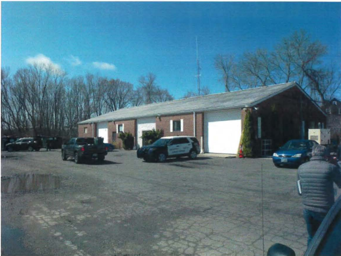
National Guard Maintenance Building – 57 Low Street
