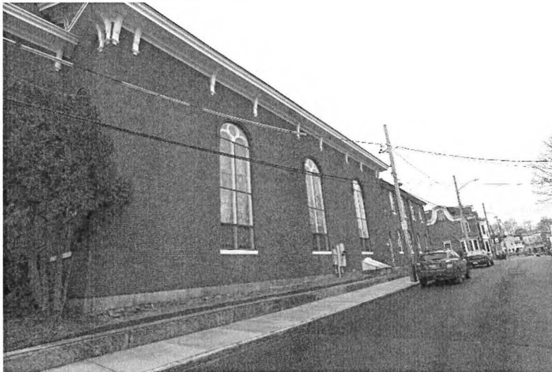
Photo 2. North Elevation, 1861 Portion, January 2020
