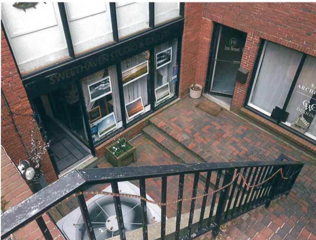
LOOKING INTO STAIRWELL FROM TOP OF STAIRS on MAIN ST.
