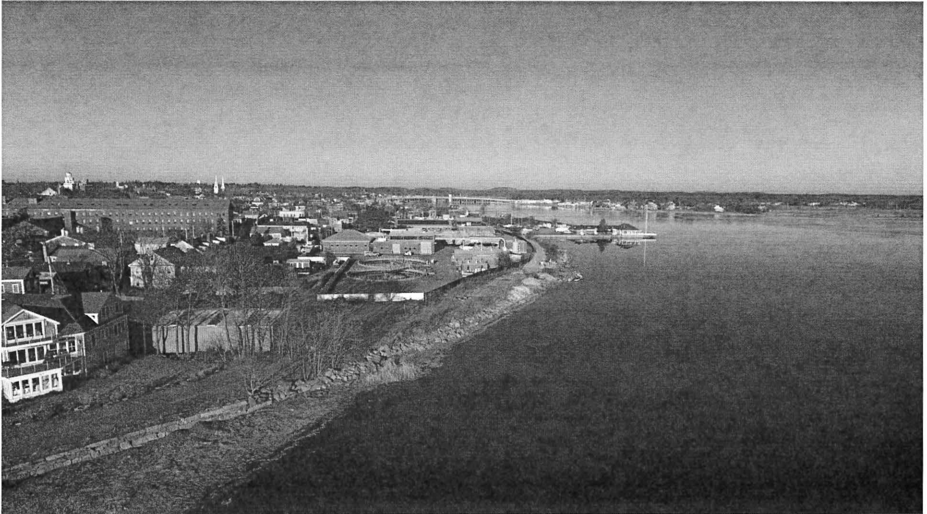
Looking northwest along old rail corridor and WWTF - note deteriorated riprap revetment and temporary shoreline stabilization
