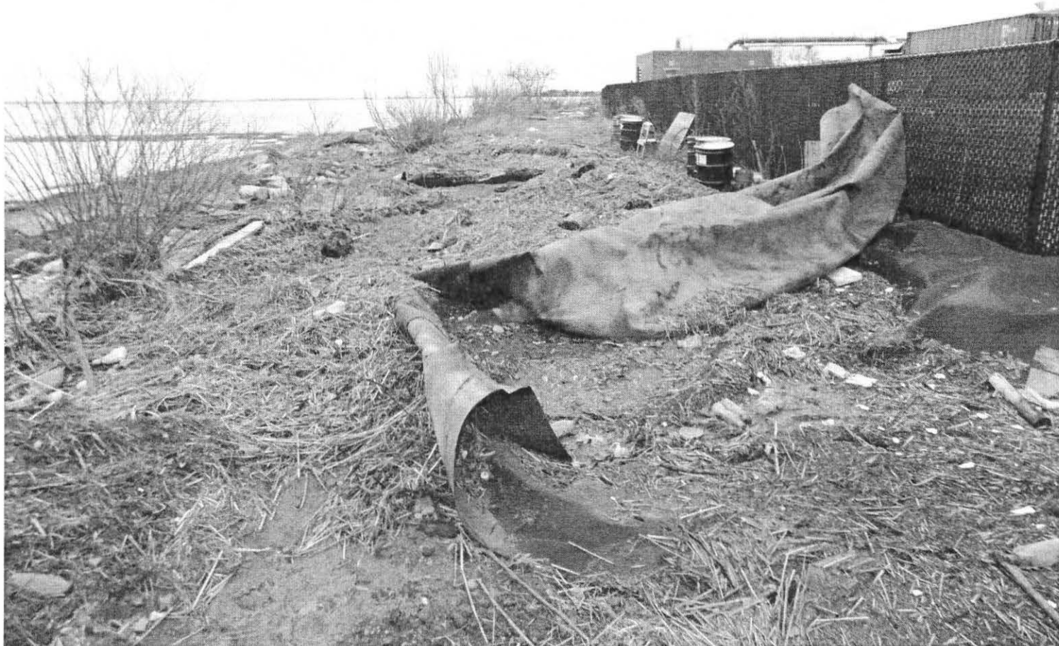
Wrack deposited from flooding across old rail corridor close to WWTF Biofilter (May 2018)
