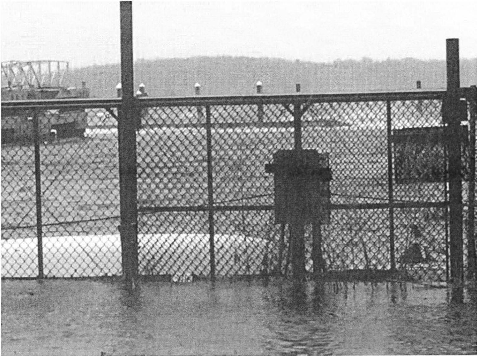
Storm surge flooding (May 2018)
