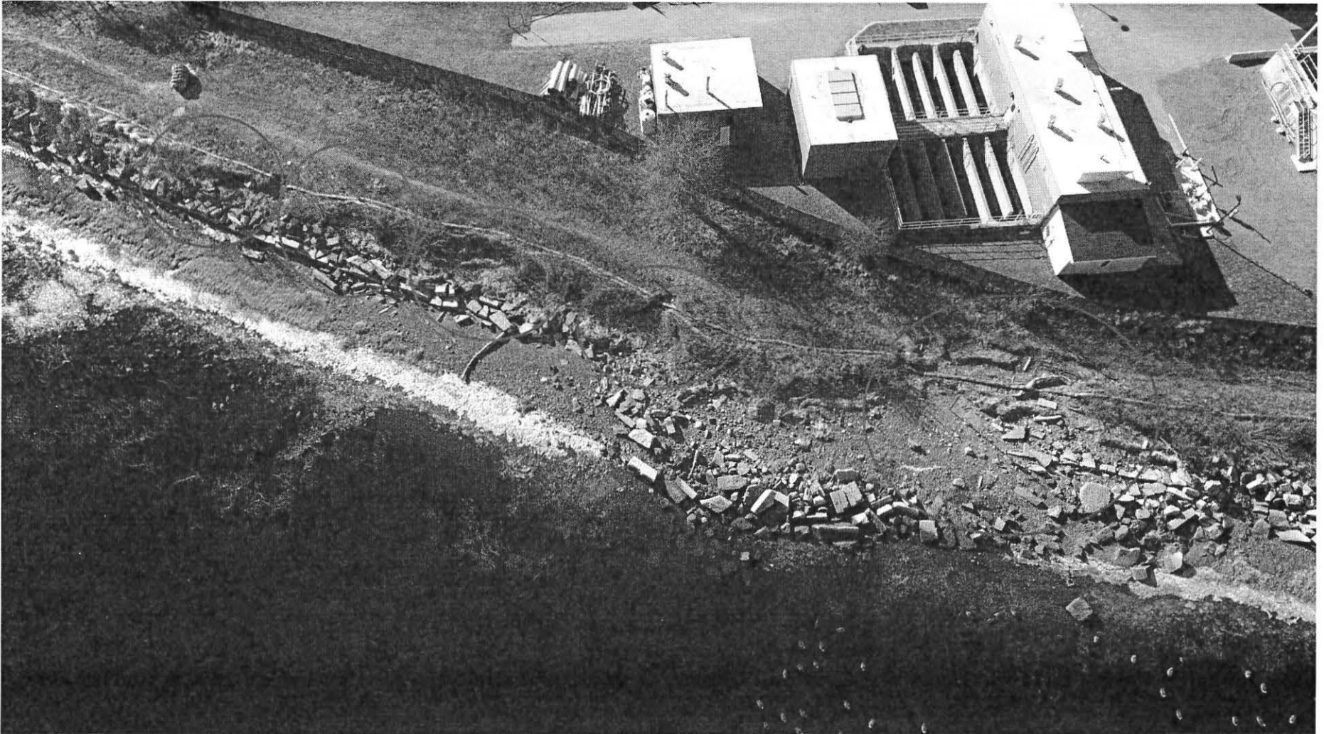
Aerial photo of part of eroded shoreline from 2018 storms – scouring into/across old rail corridor towards WWTP chlorine contact tanks (inundation at 12' flood level) and chlorination building
