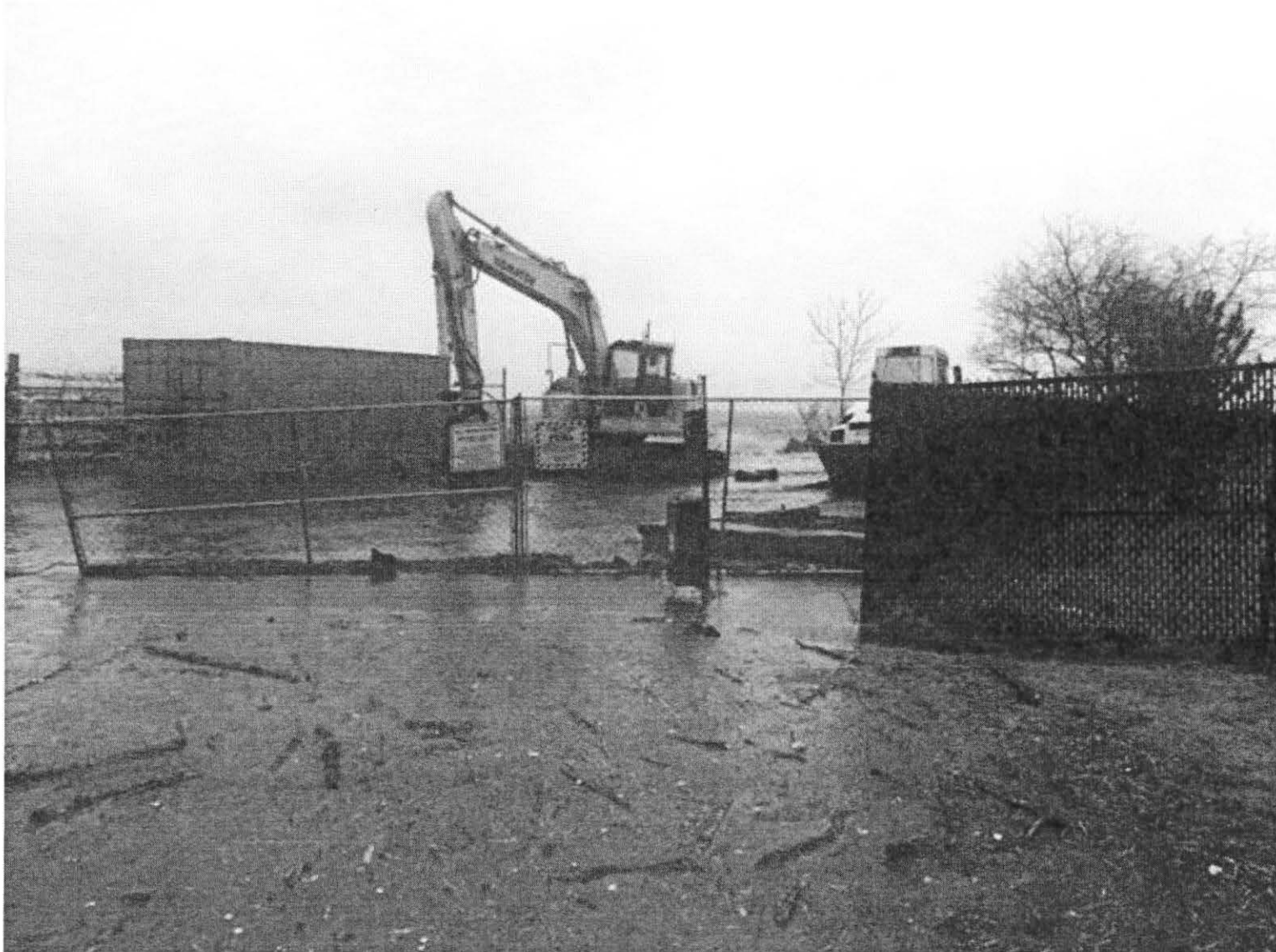
Storm surge flooding at northwest corner of WWTF (May 2018)
