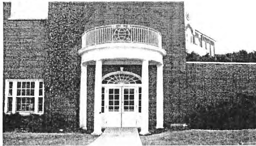
Photo 22. Northeast facade. Character defining features: arched and rectangular door surrounds with pilasters and entablatures; round window and vents with keystone details; dentil molding at cornice below parapet. April 2015.
