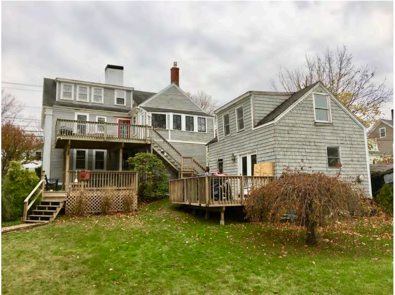
14. North Façade and Outbuilding
