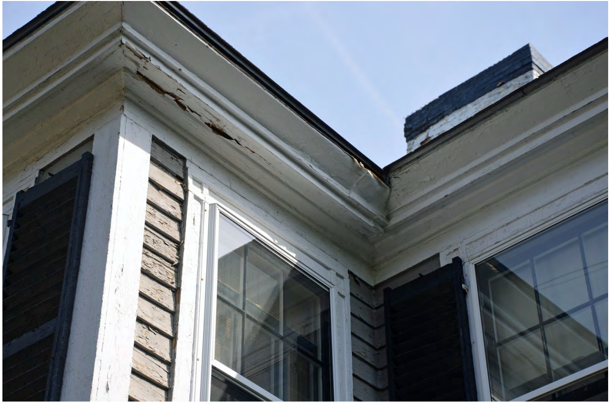
5. Fascia, Crown, Soffit, Frieze and Casing Detail
