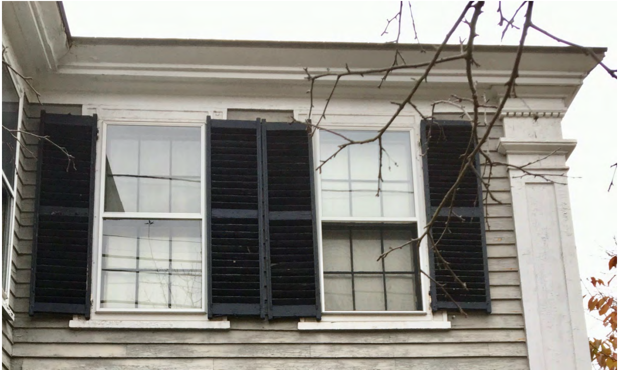
4. Fascia, Crown, Soffit, Frieze and Upper Corner Pilaster Detail
