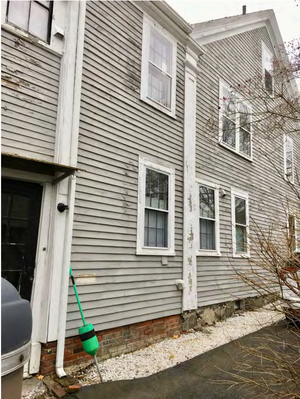
8. West Façade – Pilaster, Windows and Trim, Siding (Typ.)
