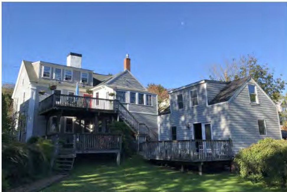
Photo 3. View of rear elevation and outbuilding, looking west.
