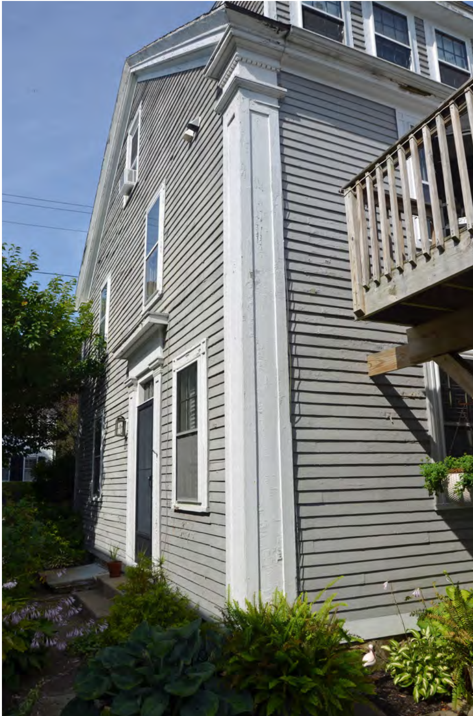
12. Corner Pilaster, Rake, Fascia and Return Detail
