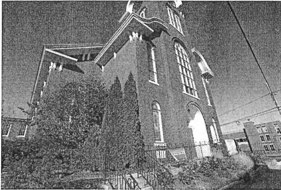
Photo 19. South and East Elevations, 1861 Portion, November 2019
