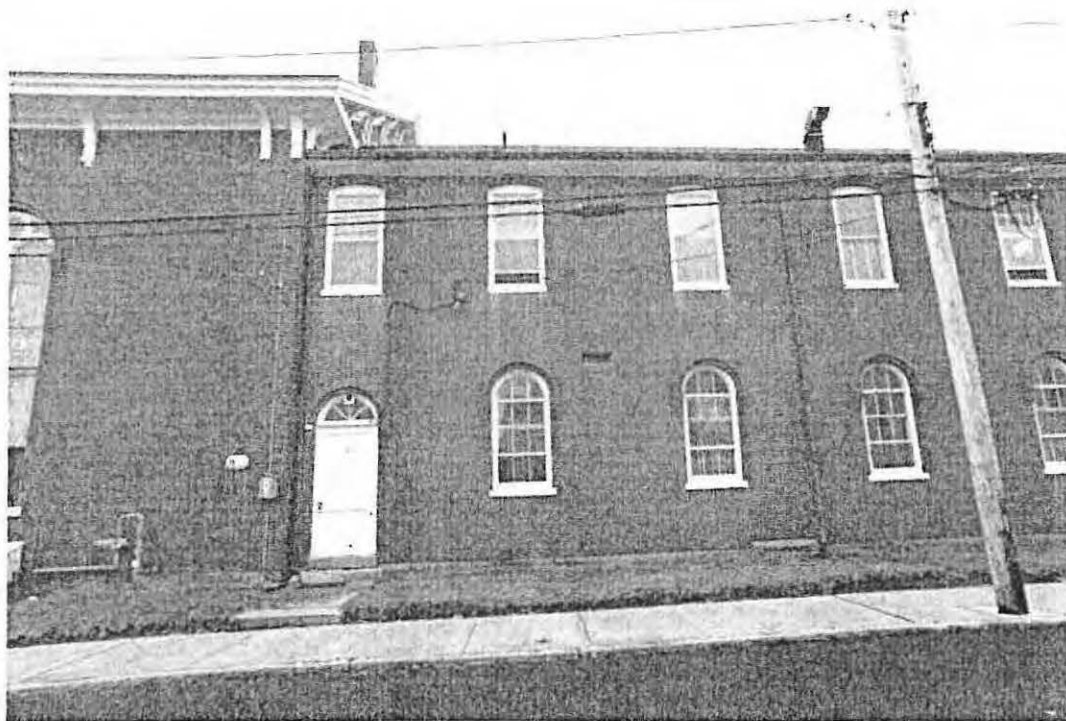
Photo 22. North Elevations, 1861 Portion and 1910 Portion, January 2020
