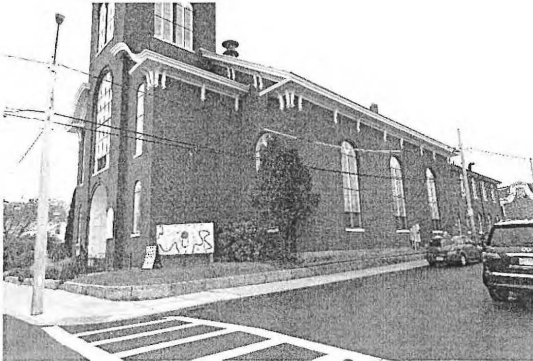
Photo 1. East and North Elevations, 1861 Portion, January 2020
