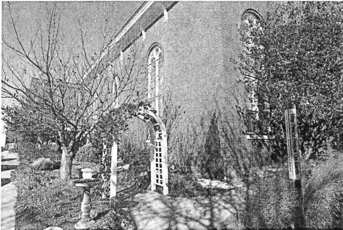
Photo 16. South and East Elevations, 1861 Portion, November 2019
