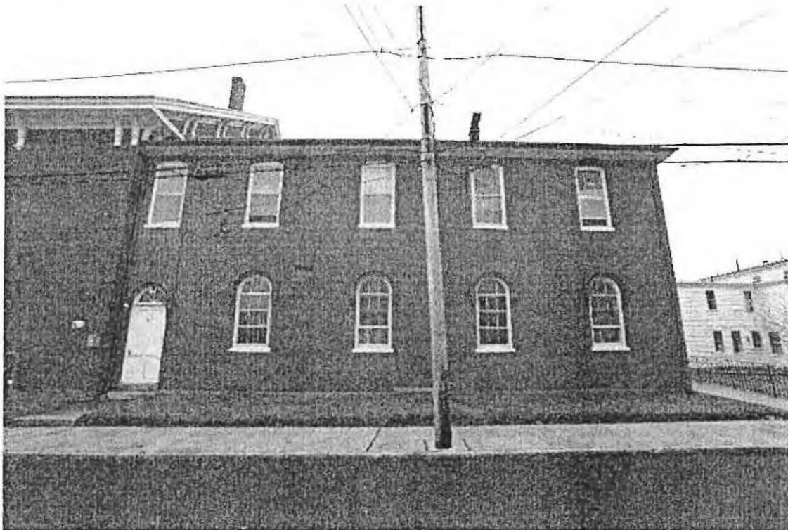
Photo 20. North Elevations, 1910 Portion and 1861 Portion, January 2020
