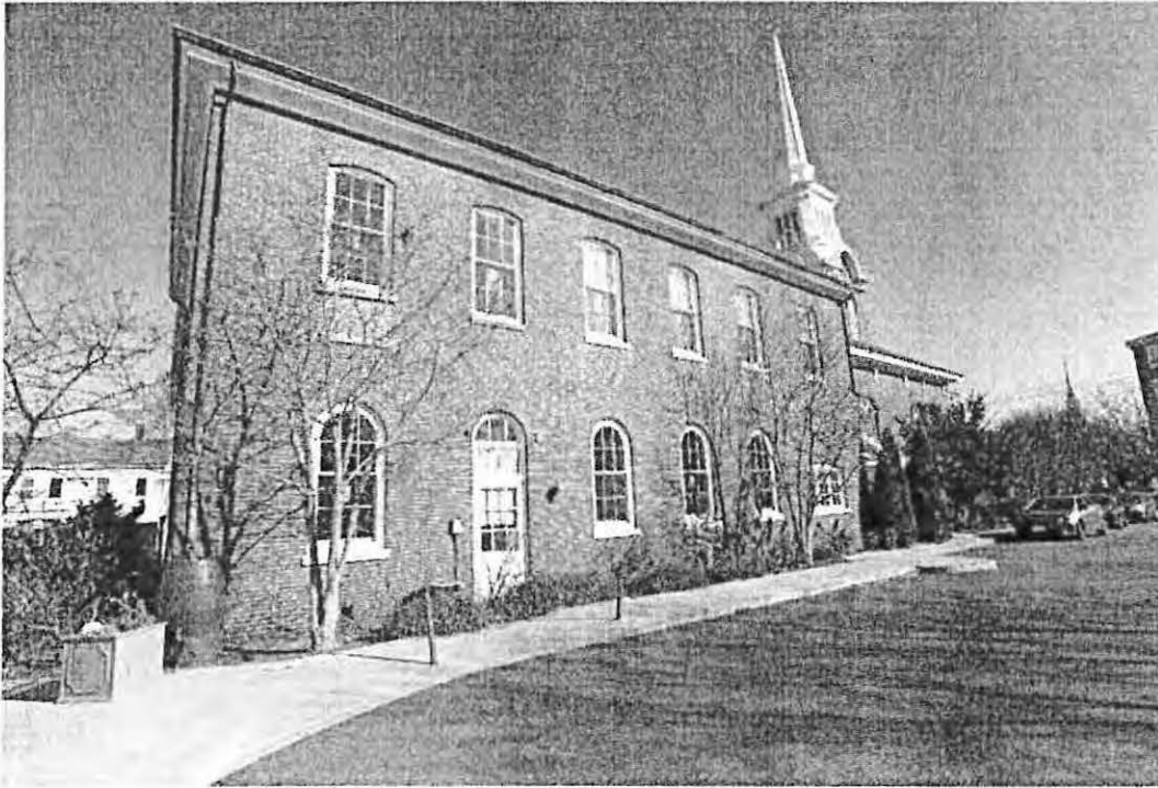
Photo 13. South Elevation, 1910 Portion, November 2019
