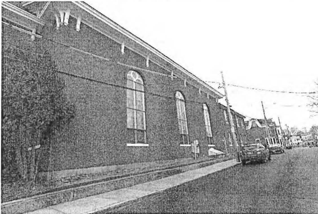
Photo 2. North Elevation, 1861 Portion, January 2020
