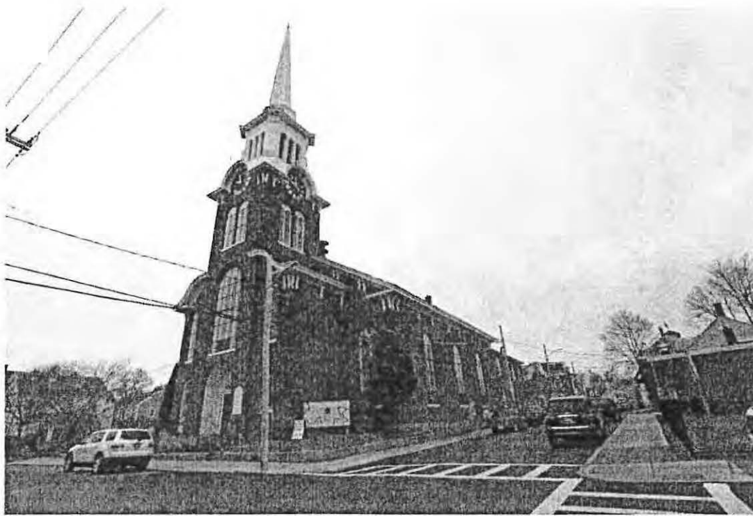
Photo 5. East and North Elevations, 1861 Portion, January 2020
