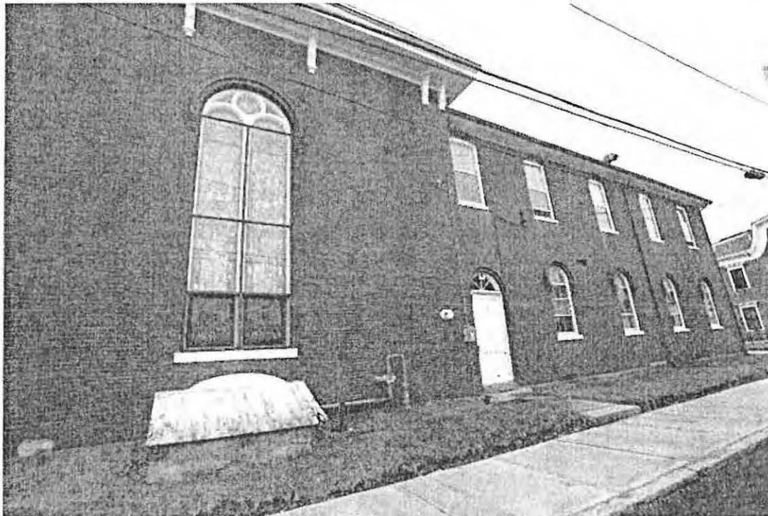
Photo 4. North Elevations, 1861 Portion and 1910 Portion, January 2020
