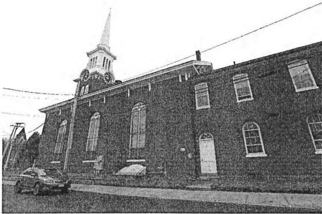
Photo 21. North Elevations, 1861 Portion and 1910 Portion, January 2020
