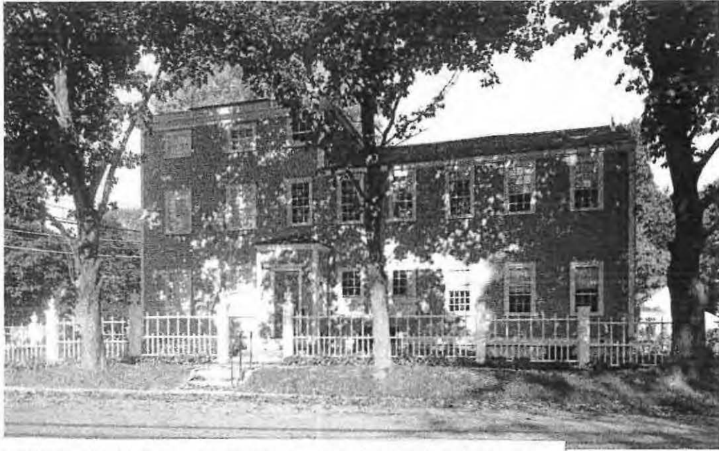
Exhibit B – MA: Newburyport, 272 High Street, THOMAS EMERY HOUSE Main Block and Rear Ell: South Elevation (neg. #56690-A)
