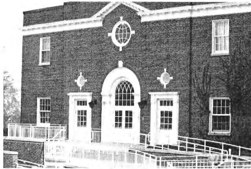
Photo 22. Northeast facade. Character defining features: arched and rectangular door surrounds with pilasters and entablatures; round window and vents with keystone details; dentil molding at cornice below parapet. April 2015.
