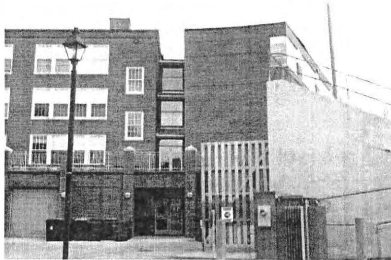
Photo 14. 2001 addition, west elevation (right). April 2015.
