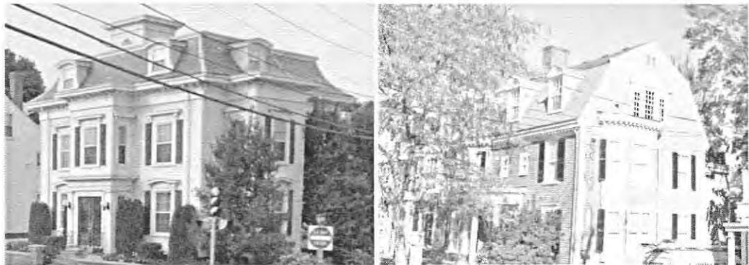
(Gabled dormers in the DOD that project from mansard and gambrel roofs.)
