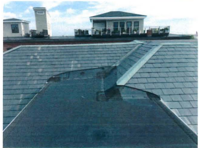
Elevator Penthouse tying into original pitched roof
