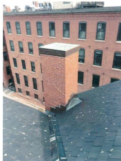
Chimney at original building with copper flashing
