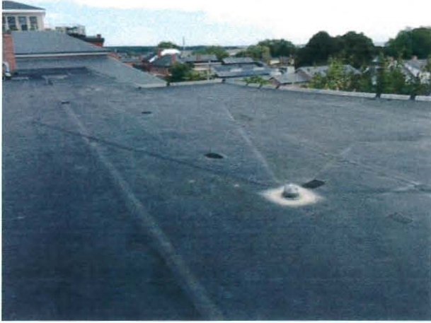
2001 Addition - Field of roof looking northeast
