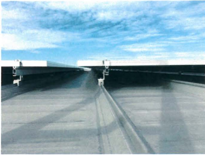
Attachment of solar photovoltaic panels on existing standing seam metal roof – minimal clearance
