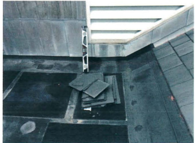
Miscellaneous slates stacked on membrane roofing
