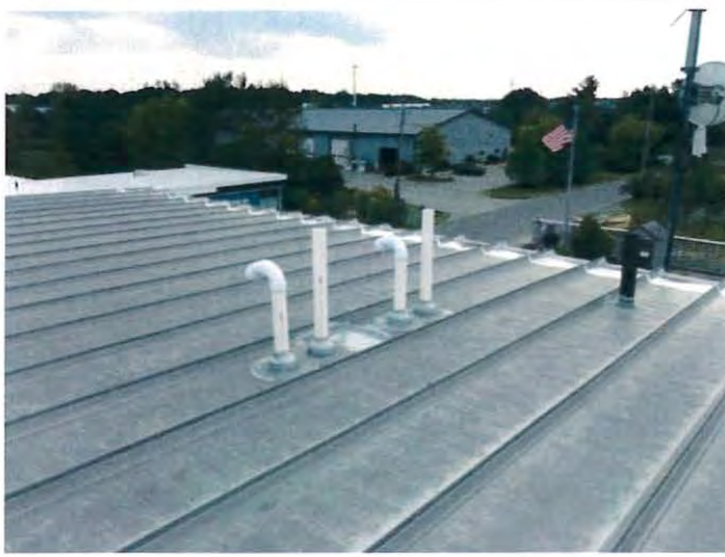
Flashing repairs at vent stacks
