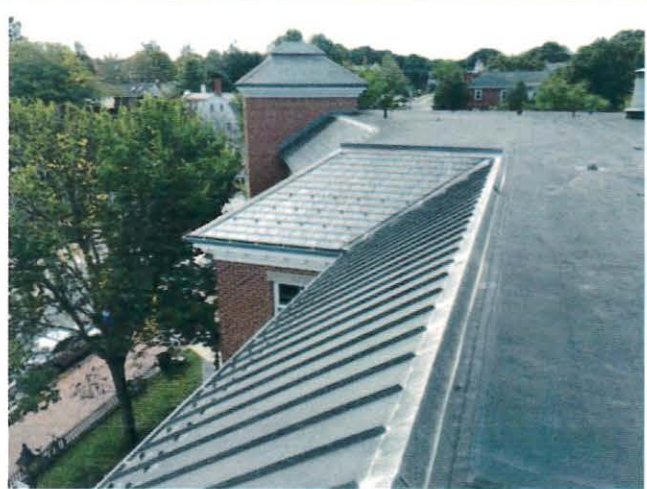
Lead coated copper standing seam roof over main entrance
