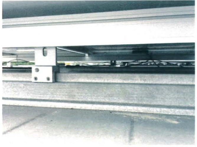
Attachment of solar photovoltaic panels on existing standing seam metal roof – minimal clearance
