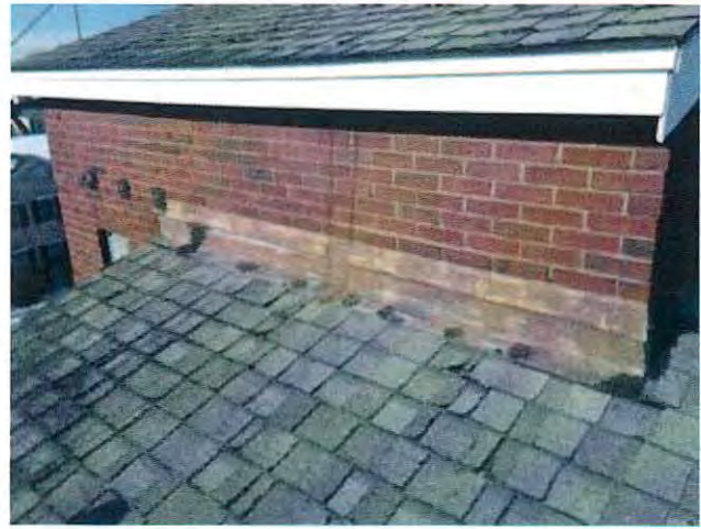
Existing copper thru-wall flashing at Hose Tower
