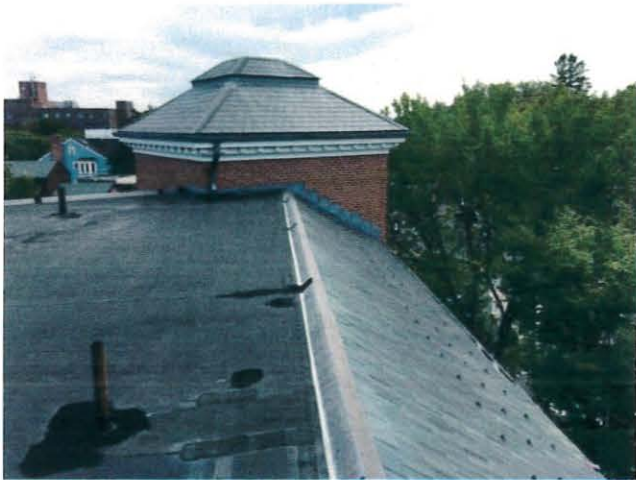
Hip slate roof tower at southeast corner of the 2001 addition
