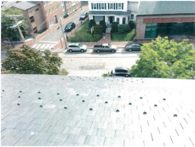
Typical snow guards, 3 rows, staggered
