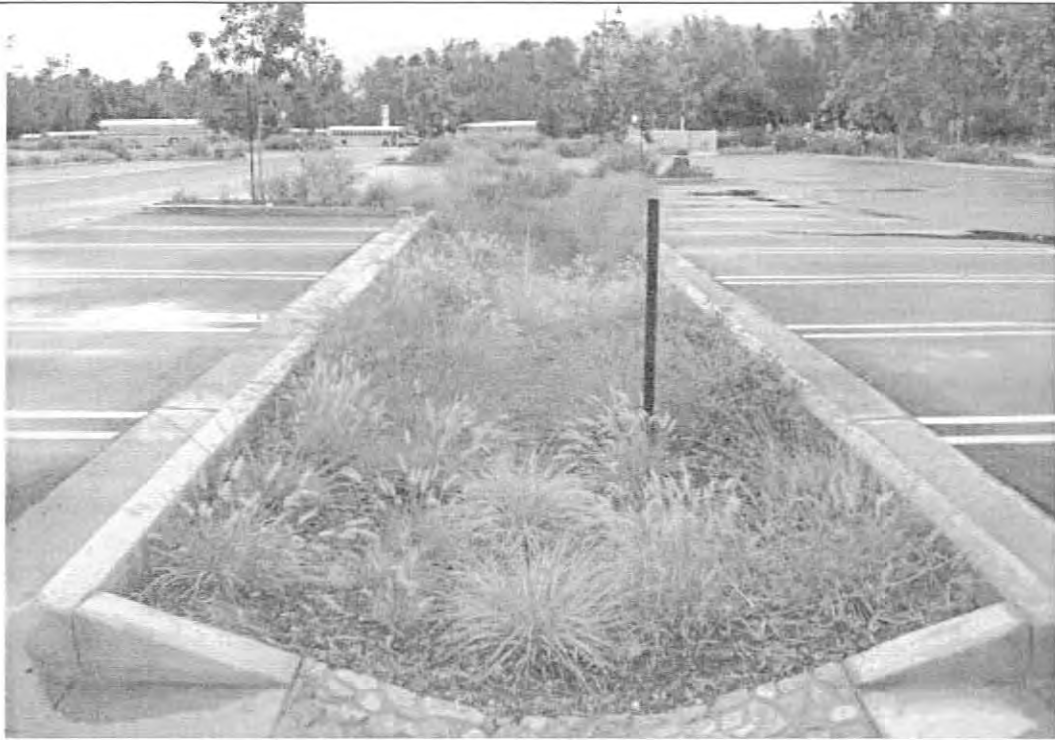
Figure 8: Attractively vegetated stormwater collection “bioretention” swales can reduce flooding and improve water quality in lieu of traditional closed-pipe drainage systems.
