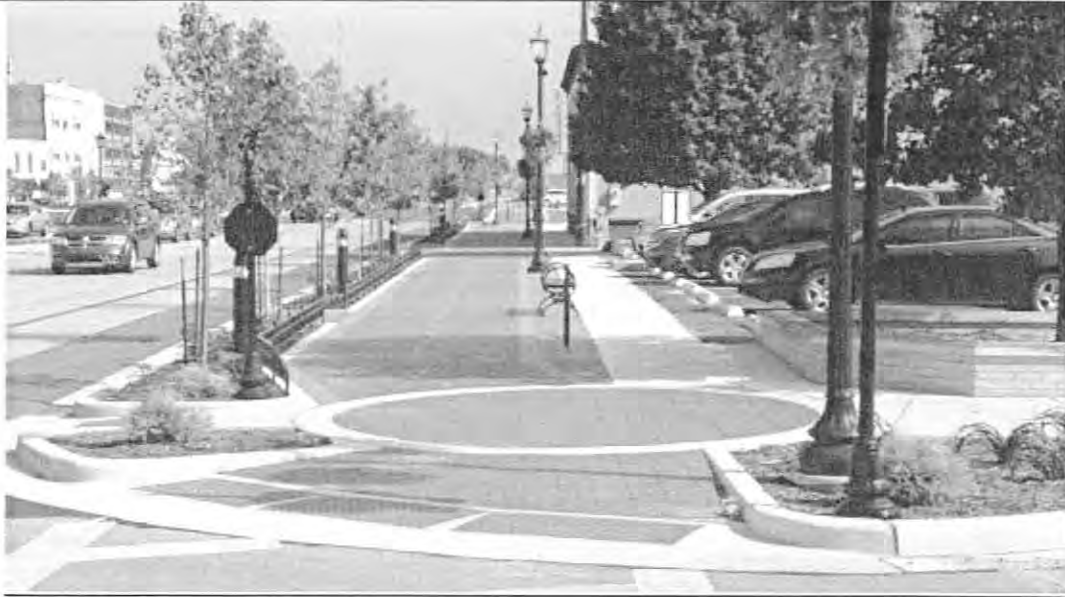
Figure 9: Changing color-coded Paver materials, landscaping, and other site amenities ensure that pedestrians know where they are safe, and advise drivers to give deference to pedestrians and bicyclists along Wharf Street, public square, and other public spaces.
