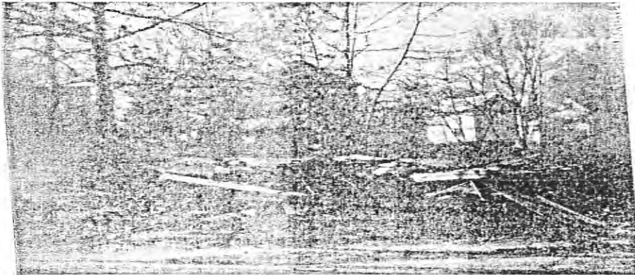
Debris piled so section between Coffin St and Jefferson St can't be used.
