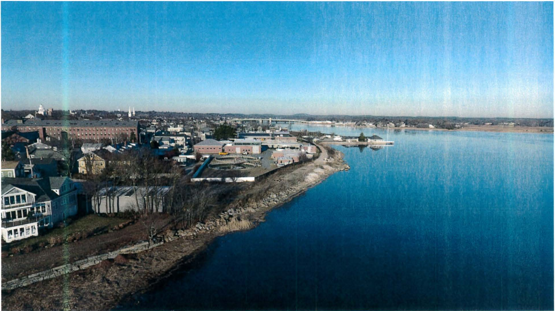
Looking northwest (December 2018) along the Merrimack River shoreline trail corridor towards downtown (note existing granite block seawall transitioning to deteriorated riprap revetment)
