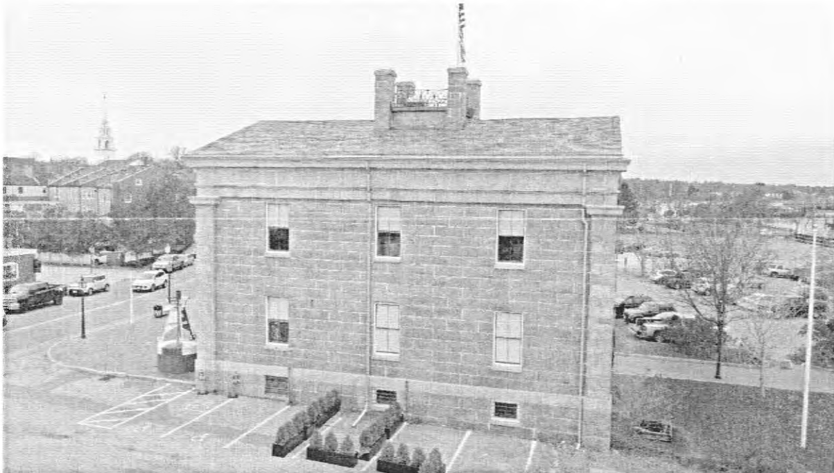
2. 11/14/2019 View of east façade, uavlook.com
