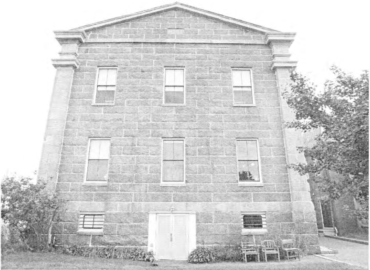
3. 7/27/2013 View of north façade, Gregory Colling
