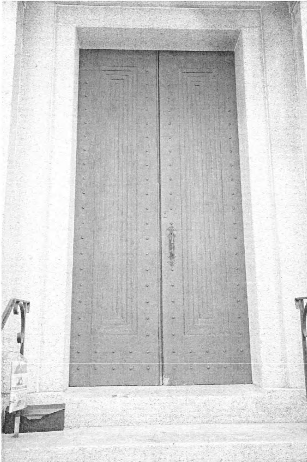
5. 3/16/2019 Water Street Entry Door Detail, Bill Finch
