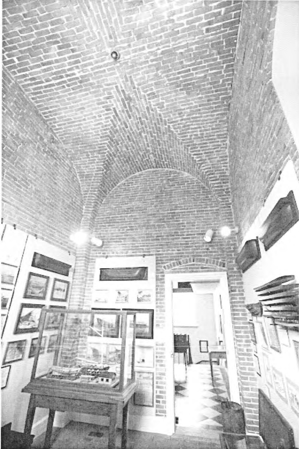
9. 6/2//2009 Second floor groin vault (Baker Gallery), Carl Tremblay
