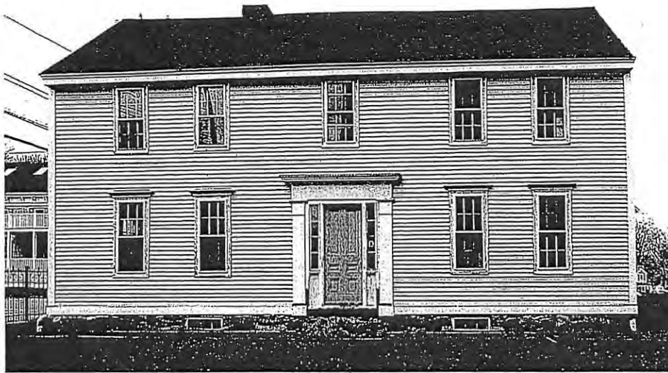
1 SOUTH ELEVATION PHOTO - 2015 N/S
