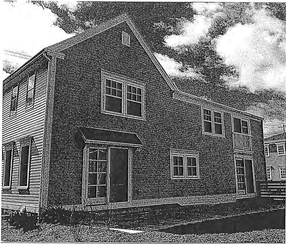
18. Rear (east) elevation – April 2017
