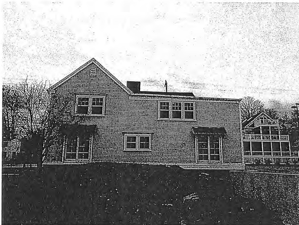
5. Rear (east) elevation – April 2015
