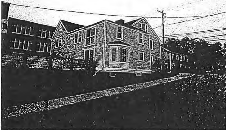
262-264 Merrimac Street, camera facing southwest
