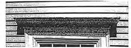
12 EXISTING WINDOW ENTABLATURE - 2017 SITE
