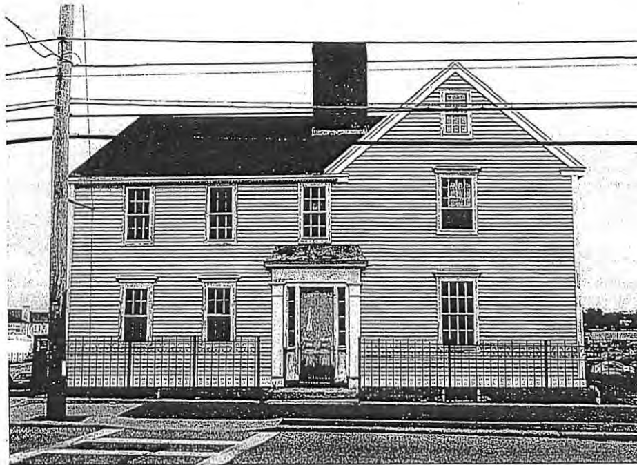
① WEST ELEVATION PHOTO - 2015 MS
