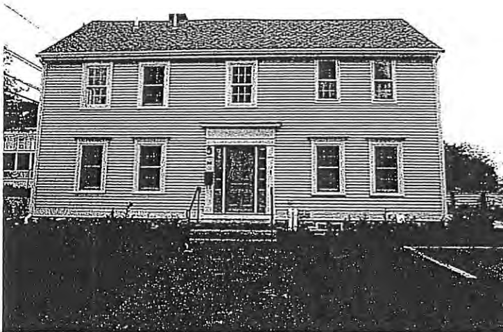
262-264 Merrimac Street, Camera facing northwest
