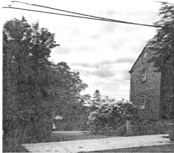
Current view from Jefferson St side
