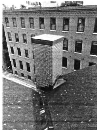
Chimney at original building with copper flashing
