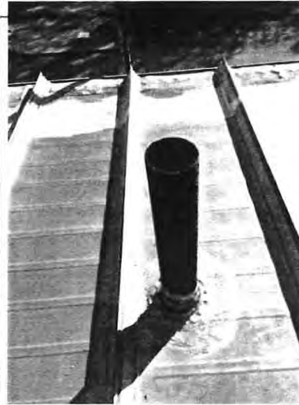
Dek-Tite pipe flashing poorly installed - missing stainless steel clamps, fasteners, and mastic repairs
