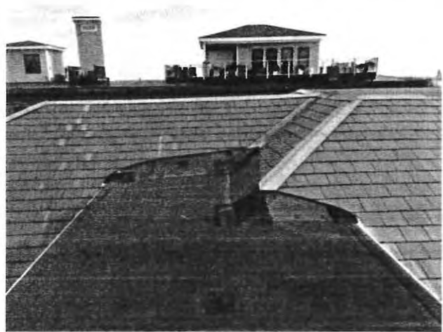
Elevator Penthouse tying into original pitched roof
