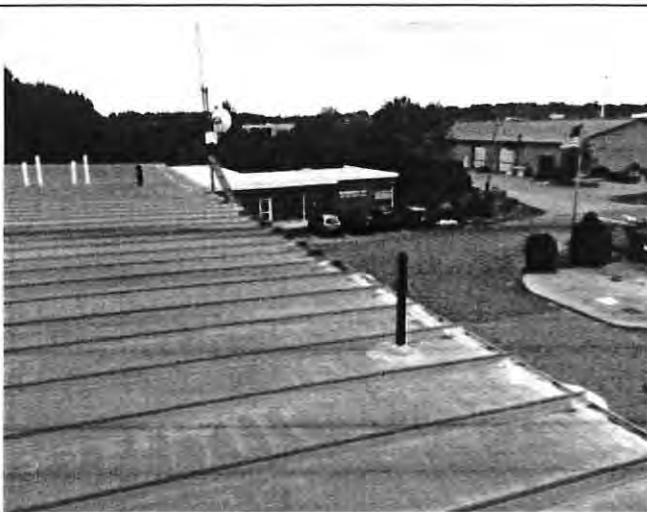
Overview looking east
