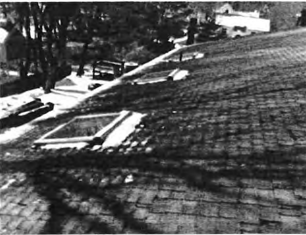
Skylights at the rear of the building
