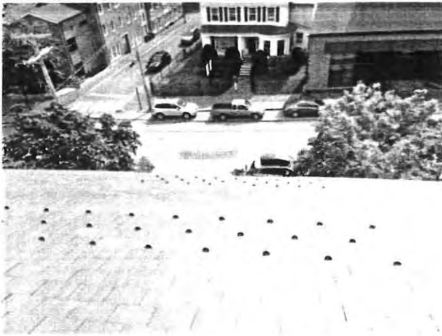
Typical snow guards, 3 rows, staggered
