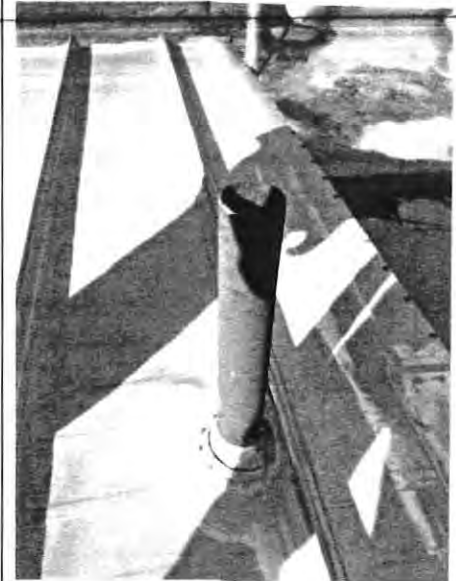
Dek-Tite pipe flashing poorly installed - missing stainless steel clamps, fasteners, and mastic repairs
