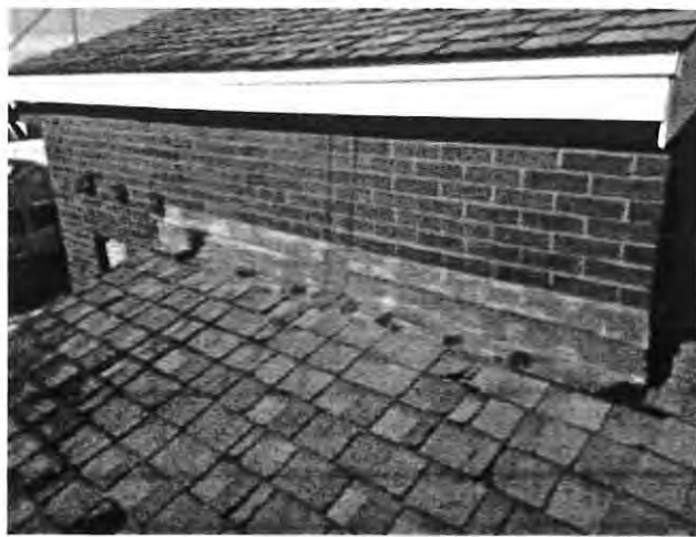
Existing copper thru-wall flashing at Hose Tower
