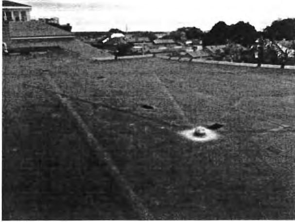
2001 Addition - Field of roof looking northeast
