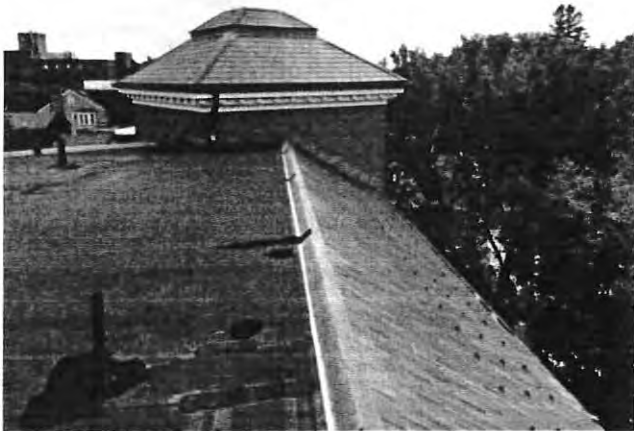
Hip slate roof tower at southeast corner of the 2001 addition
