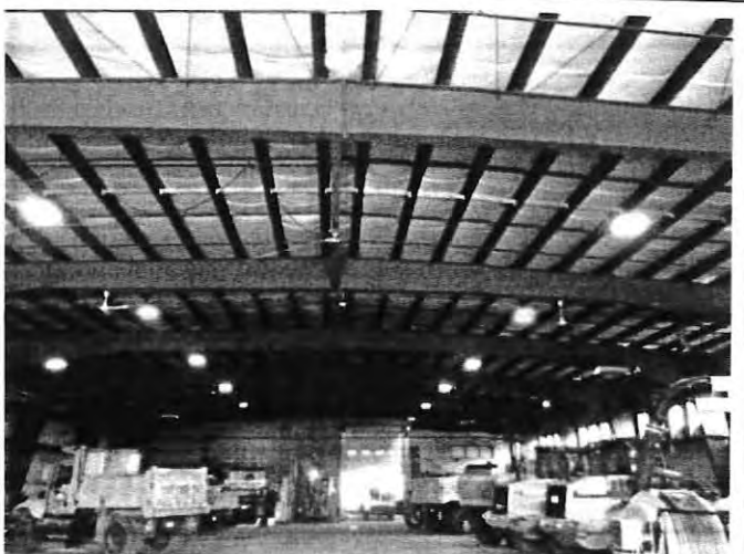
Interior steel frame with insulation blankets at roof purlins
