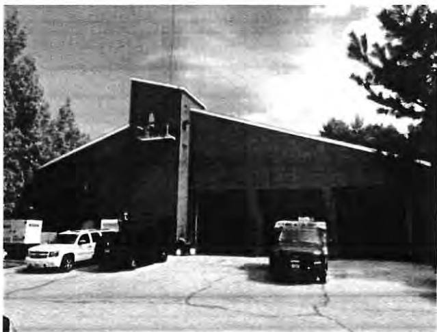
Overview - west side
