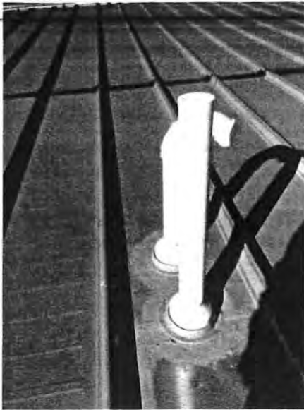
Dek-Tite pipe flashing poorly installed - missing stainless steel clamps, fasteners, and mastic repairs
