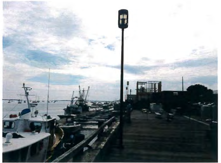
Looking east from boardwalk towards building
