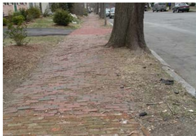
Figure 106. Compromised Sidewalks
