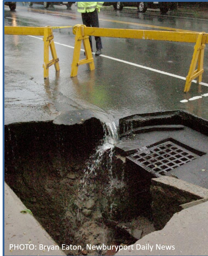
Figure 108. Storm Drain Sinkhole - Created by Heavy Rains
