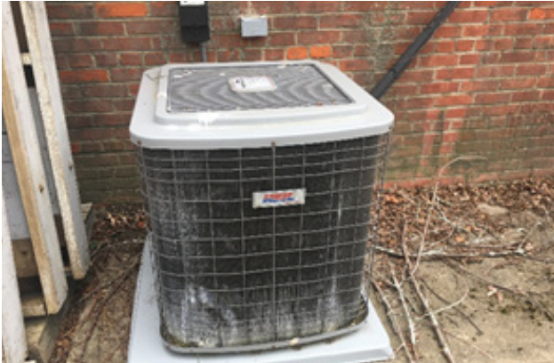
Existing Air Cooled Condensing Units
