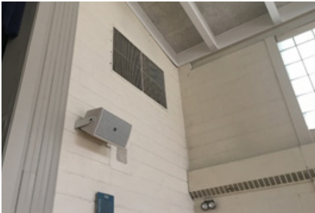
Gym - Wall Supply Diffuser + Radiation Heating
