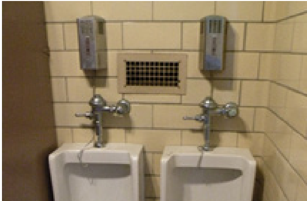
Ground Level Toilet Room - Exhaust Grille
