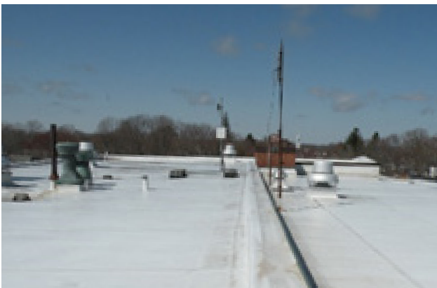
Roof Exhaust + Ventilators
