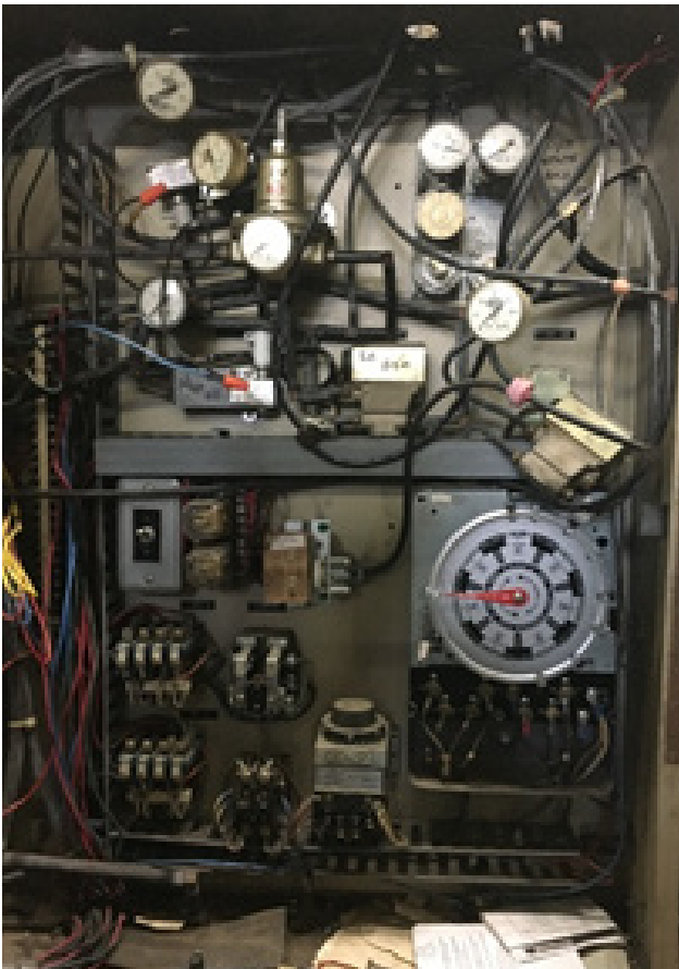
Existing ACT Pneumatic Control Panel
