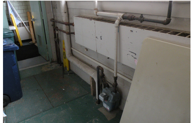
Ground Level Storage Room - Fin Tube Radiator
