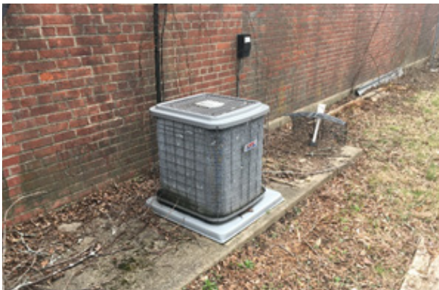
Existing Air Cooled Condensing Units
