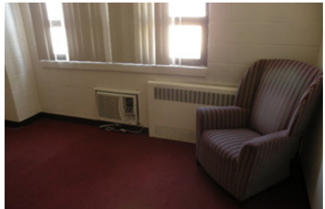
Second Floor Administration Office - Window AC / HW Convactor
