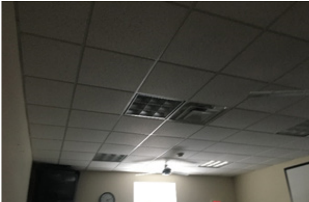
Office Ceiling Supply Diffuser + Paddle Type Fan
