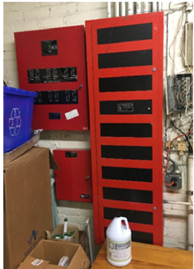
Fire Alarm Control Panel
