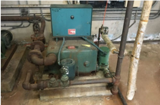
Existing Condensate Pump
