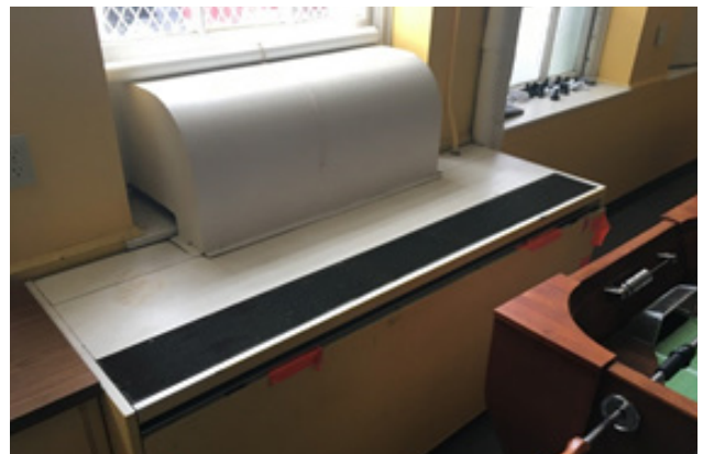
Ground Level Classroom Unit Ventilator
