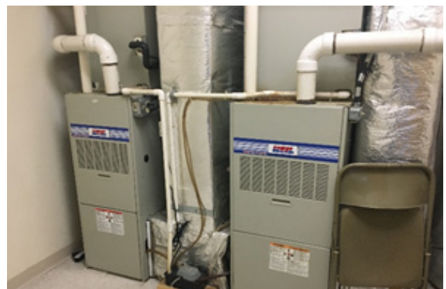
Existing Gas Fired Furnaces
