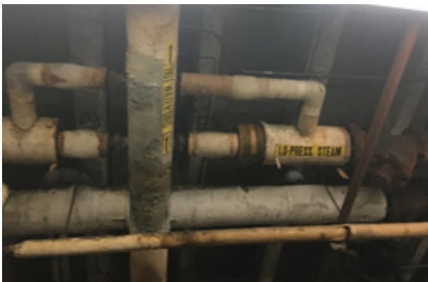
Existing Hot Water + Steam Piping
