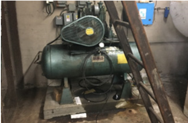
Existing ATC Compressor + Dryer
