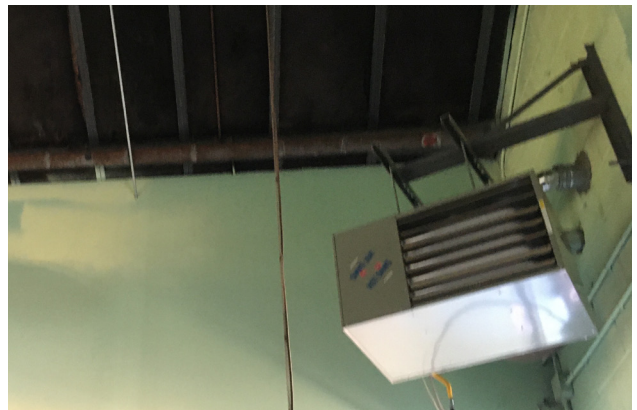
Gas Fired Unit Heater
