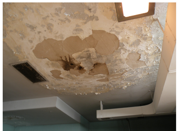
Moisture damage in the ceiling
