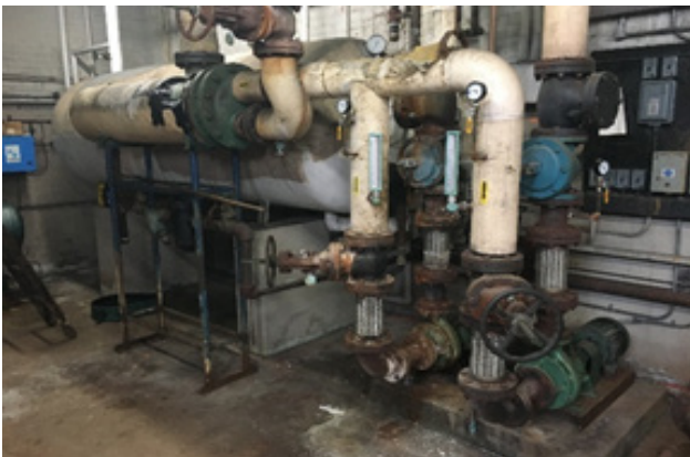
Existing Heat Exchangers + Pumps
