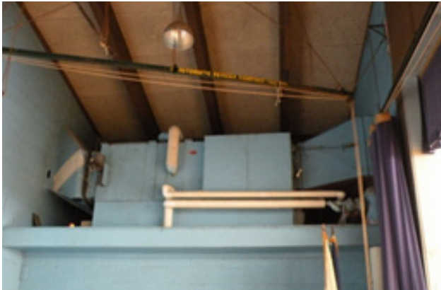
Gym - Heating + Ventilation Unit
