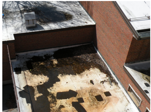
Roof over boiler room needs better drainage
