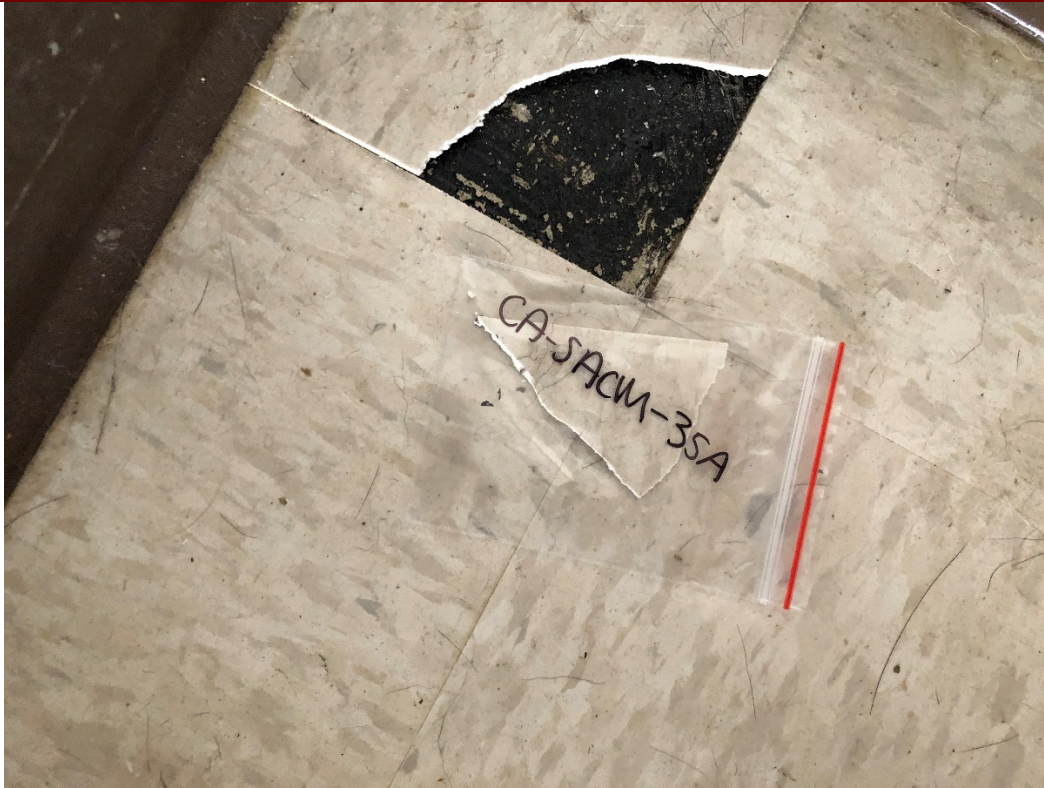
27. View of CA-SACM-34, 12" x 12" floor tile, white (sample mis-labelled in field) (Room M1-1)
