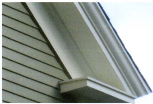
Photo 8: Preserved rake and bed moulding
