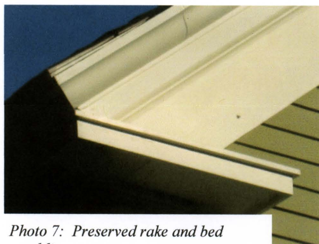
Photo 8: Preserved rake and bed moulding
