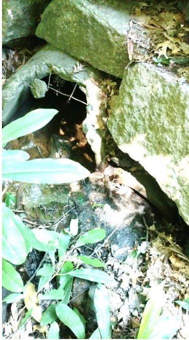
Picture 2: Two outlet pipes downstream of the road/berm. Pipe to right completely clogged.
