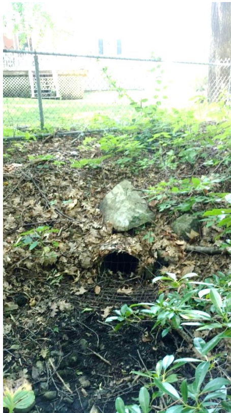
Picture 3: Inlet of 12" pipe behind 37 Phillips Drive. This pipe collects all the discharge flows from Cherry Hill's detention pond RES 10.
