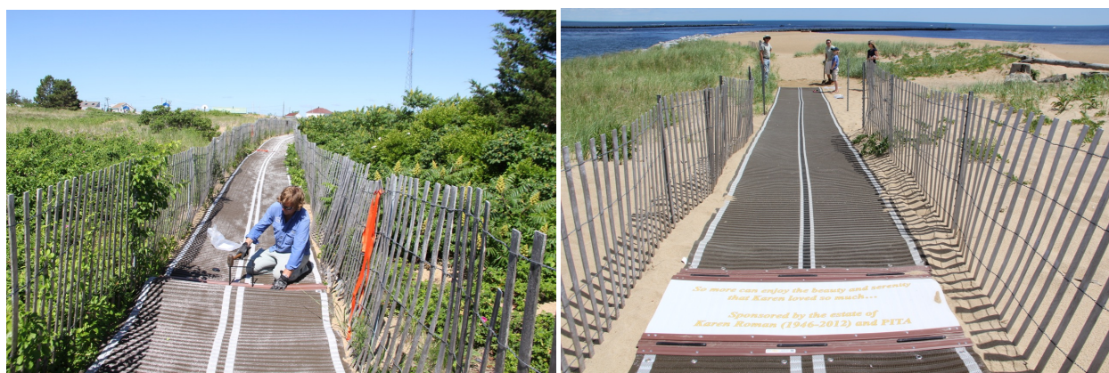
Figure 5. Installation of Mobi-Mats® on Trail 2 (left) and Trail 7 (right) required considerable effort to follow the natural meanders of the existing beach access ways, but provides full access from road to beach for all beachgoers.
