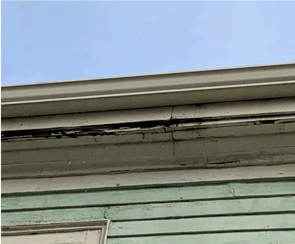
Figure 8A – Soffit and Trim Repair
