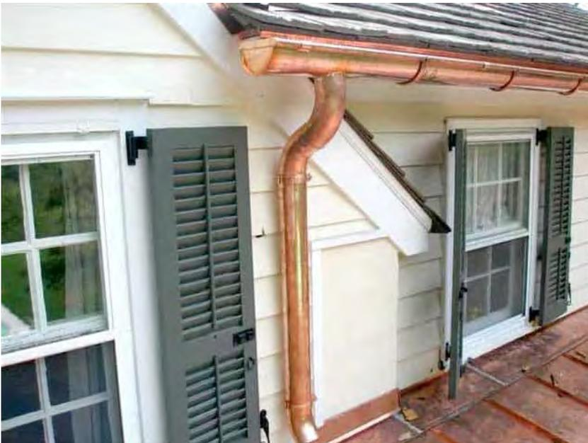
*Figure 7 – Examples of Gutters and Downspouts*
