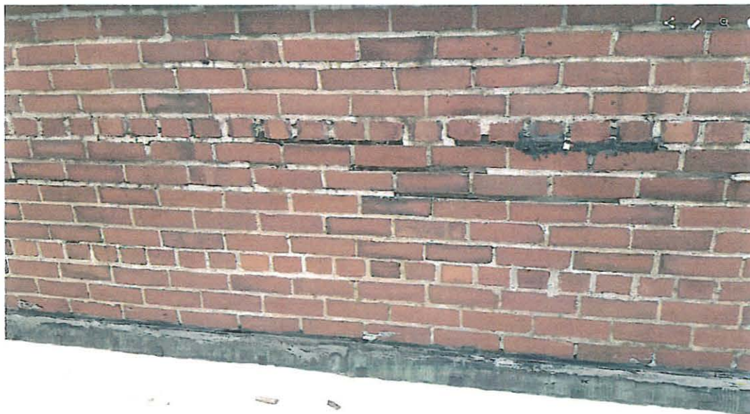
Auditorium Roof Section: Photo shows section of rising wall above roof that needs repointing
