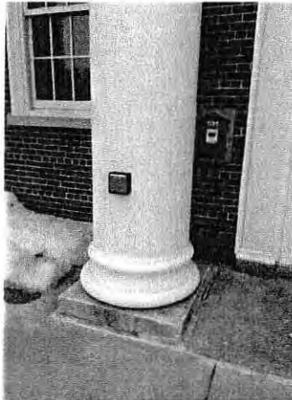
Main Entry Handicap Operator Push Button
