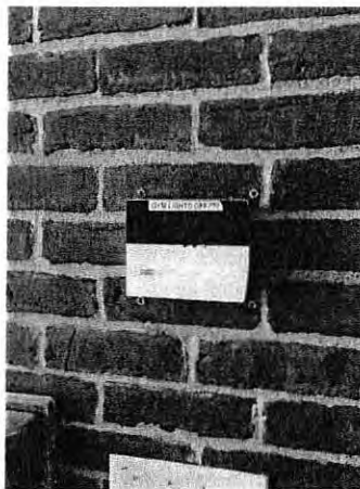
Existing Intrusion Alarm Keypad
