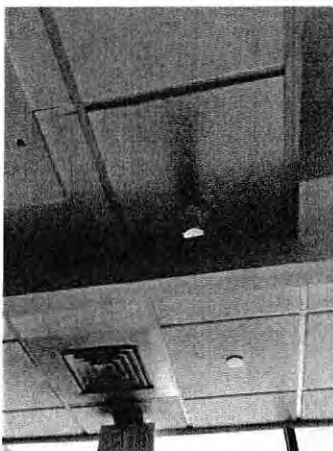
Existing Intrusion Motion Sensor
