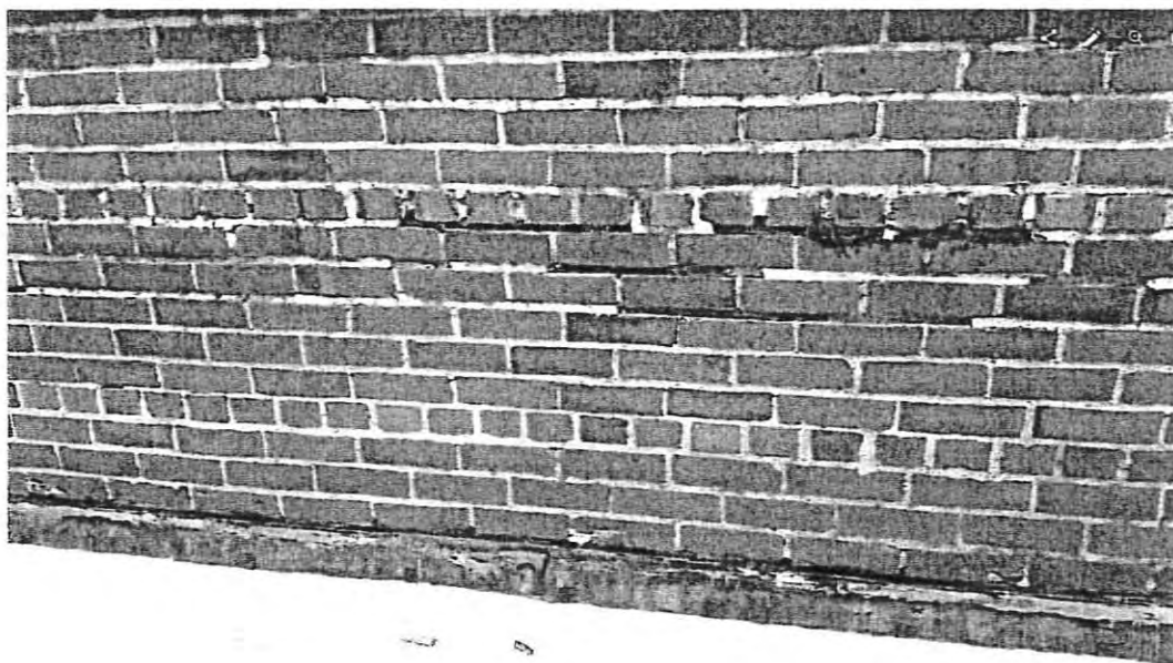
Auditorium Roof Section: Photo shows section of rising wall above roof that needs repointing
