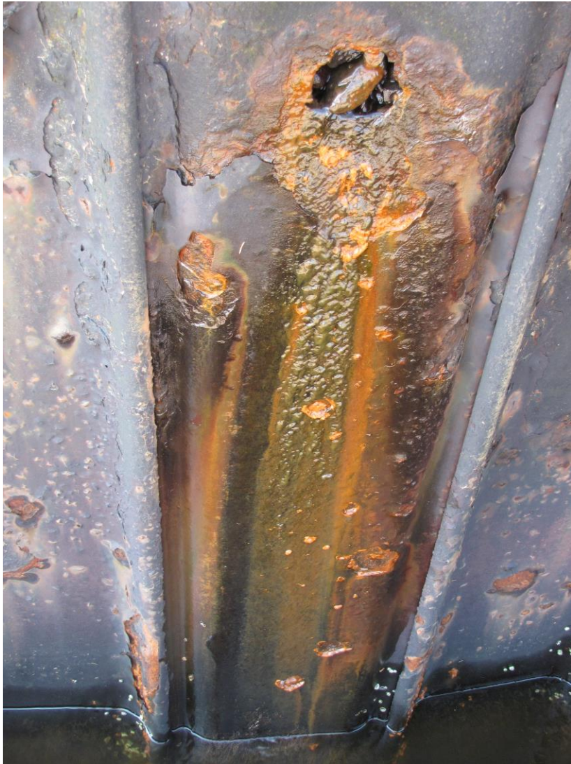
2013 typical conditions: corroding weep hole
