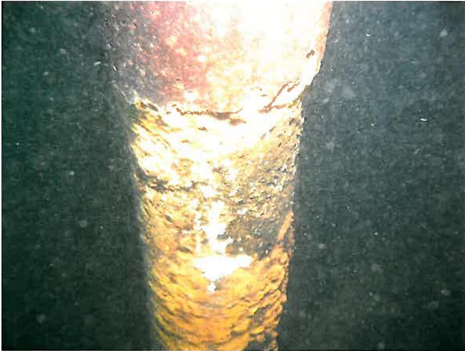
Mooring piling underwater – loss of steel and exposed concrete
