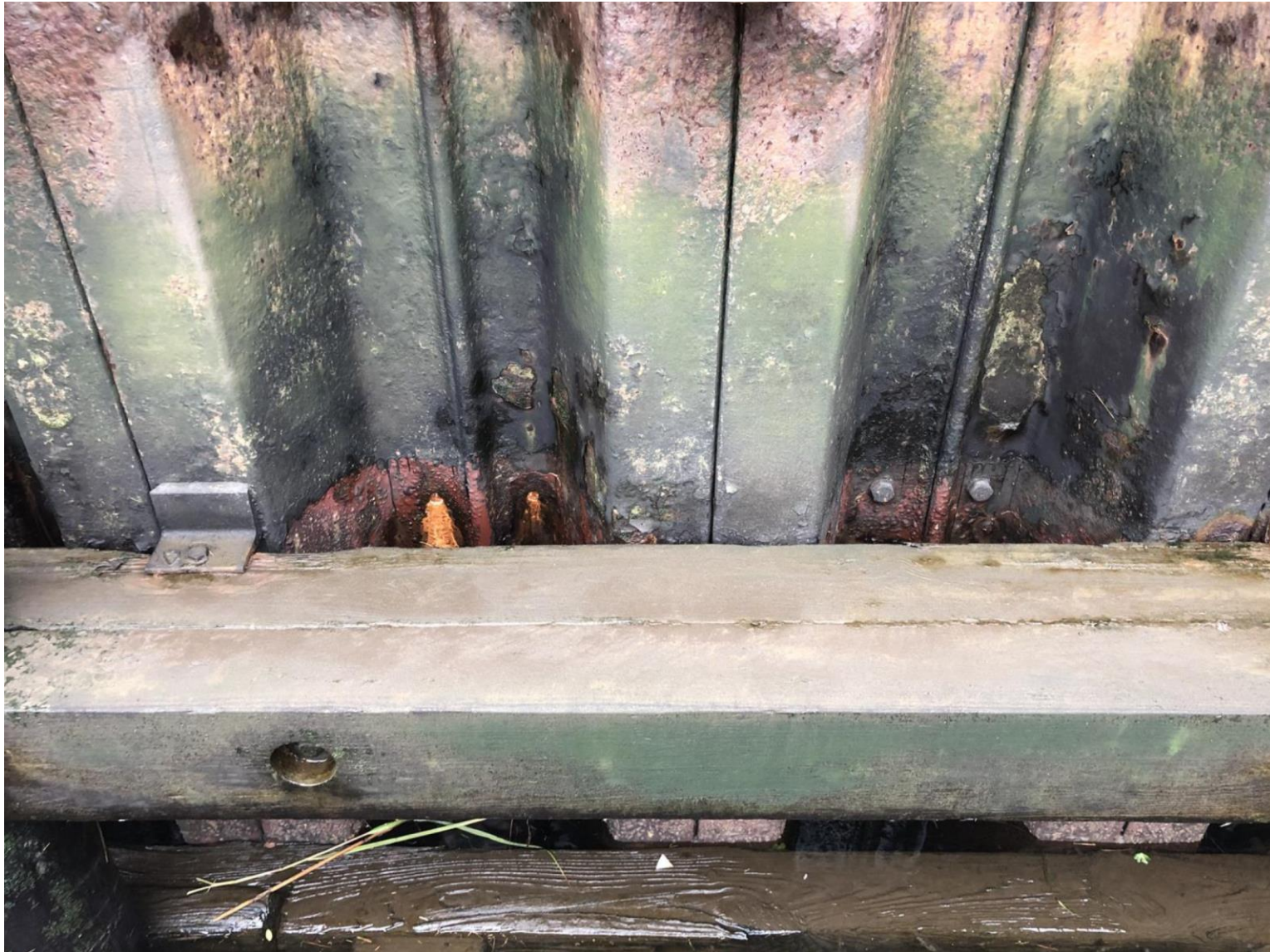
Failing Tie Back Anchor Bolts – Structural Concern
