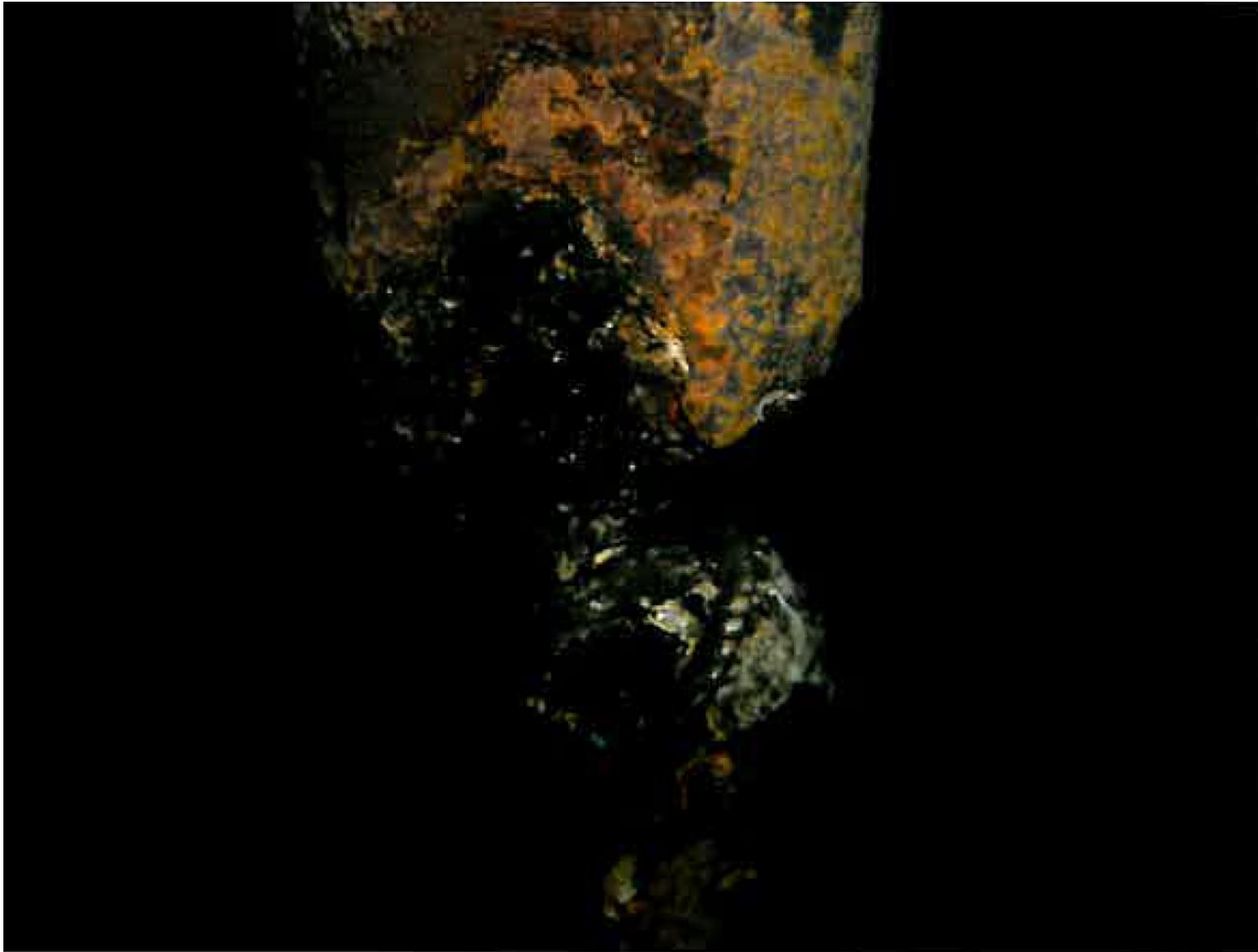
Mooring piling underwater – no steel remaining and loss of concrete fill
