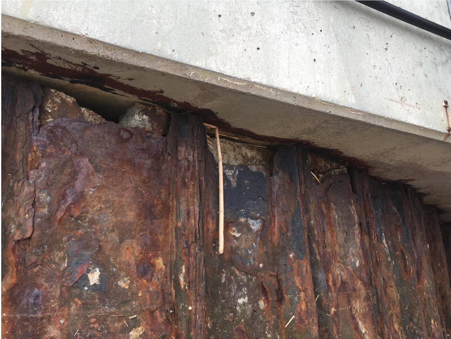
Splash zone steel section loss - loss of fill behind bulkhead
