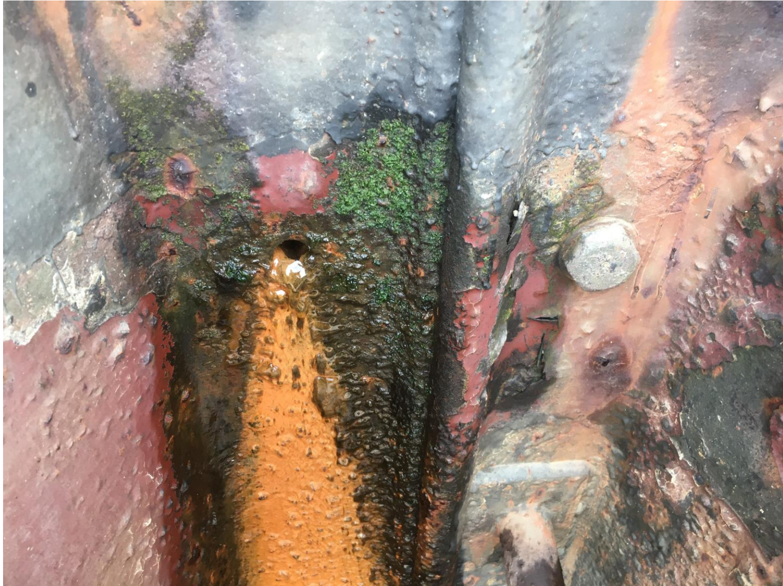
Failing Tie Back Anchor Bolts – Structural Concern
