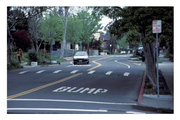
These devices reduce speed by introducing modest up-and-down changes in the level of the street, thereby requiring drivers to decelerate.
