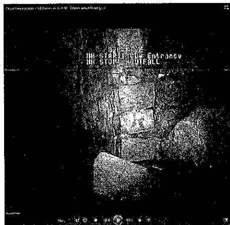
CAMERA IN CULVERT AT BASE OF CATCH BASIN, LOOKING TOWARDS THE RIVER. THE BRICK AND STONES BEHIND BRICK IS ESSENTIALLY THE CATCH BASIN – CULVERT TO THE LEFT, BASIN TO THE RIGHT – LARGE VOIDS FROM WASHOUT.
