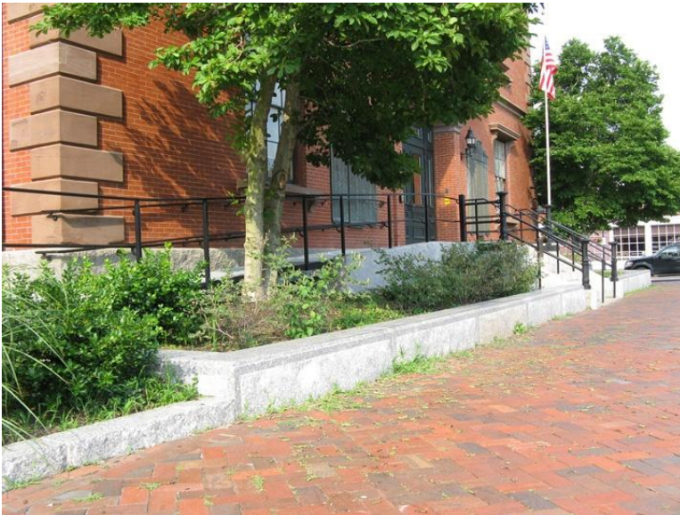
Well-designed accessible entrance ramp at City Hall.
