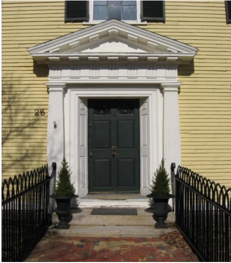
Late Georgian period door surround.
