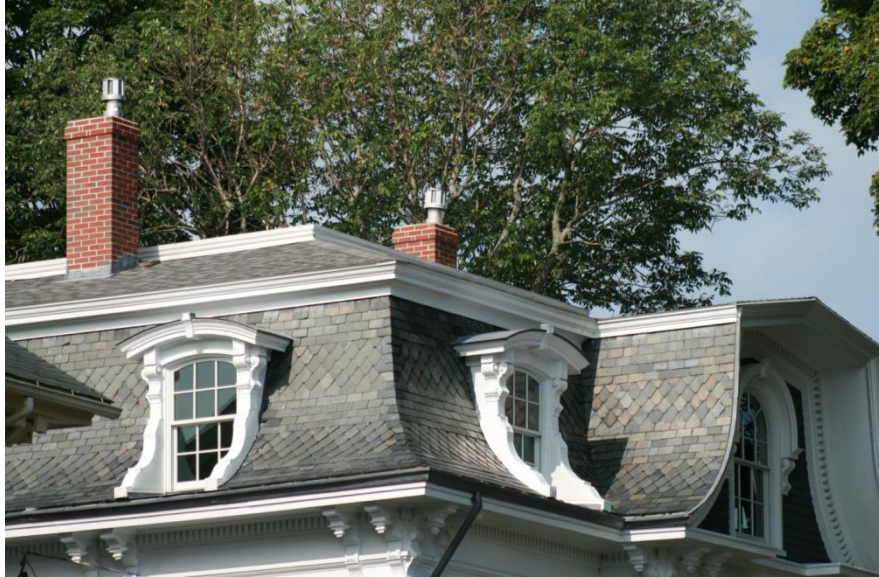
Mansard roof typical of Victorian period with decorative slate roof.
