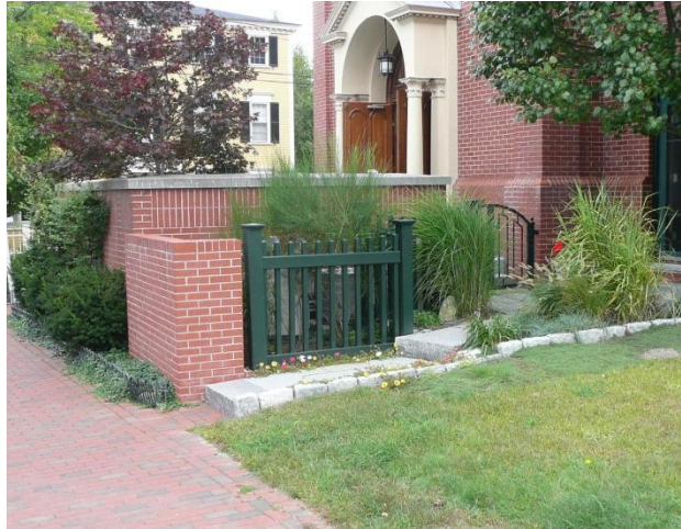
Screened mechanical equipment.
