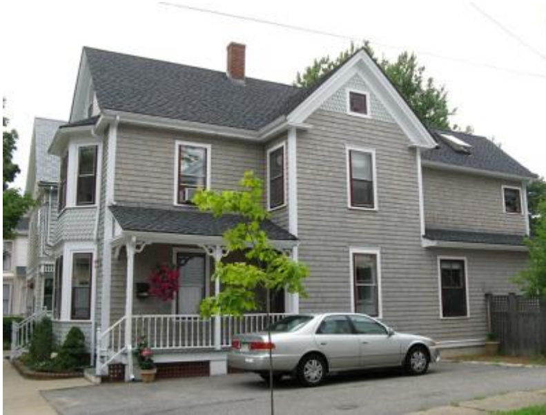
New back addition relating to the older main structure.
