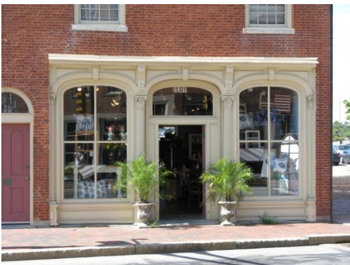
Cast iron storefront with entry flanked by display windows.
